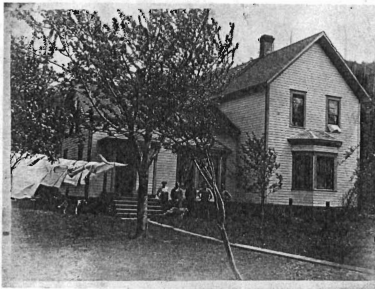
VIEW OF THE BACK OF THE ROBERTS' HOUSE
