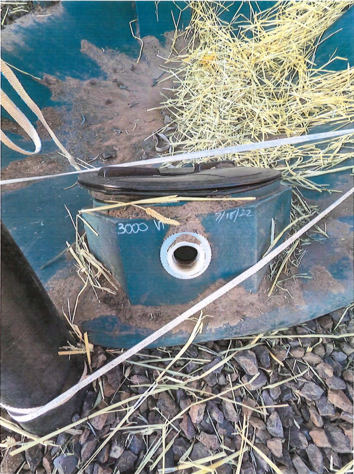
Below photo of installed pump vault/tank with pipeline connection to reservoir, top of tank and lid observed, photo from November 21, 2022 taken by Jim Newton, CWRE, of Cascade Geoengineering, LLC.
