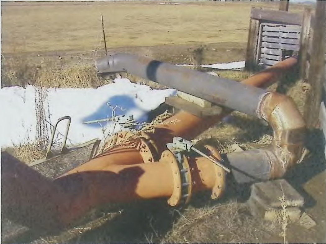
10" open discharge to the USBR C-4-C lateral.
