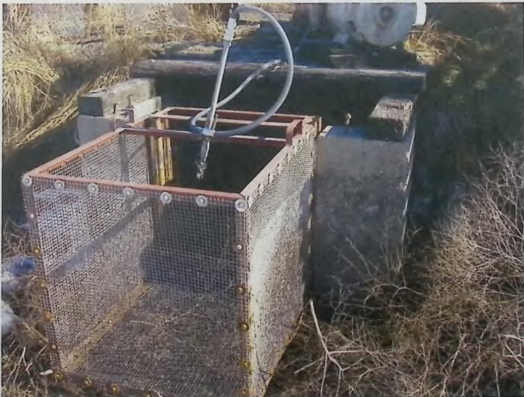
Intake in the USBR C-4-C lateral with screening, at 50hp motor and pump.
