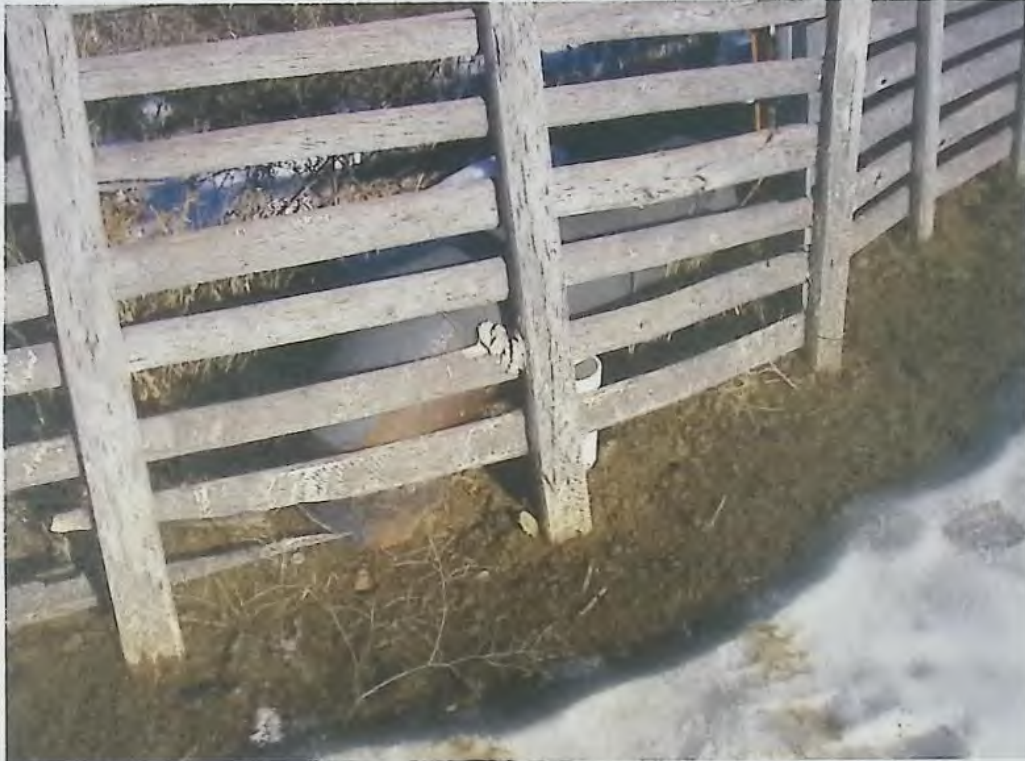
12" steel main surfacing from underground.
