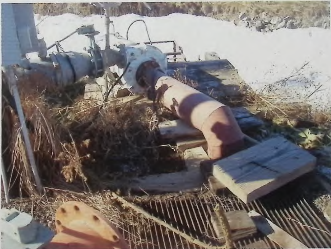
50hp booster pump currently connected to USBR C-4-C lateral
