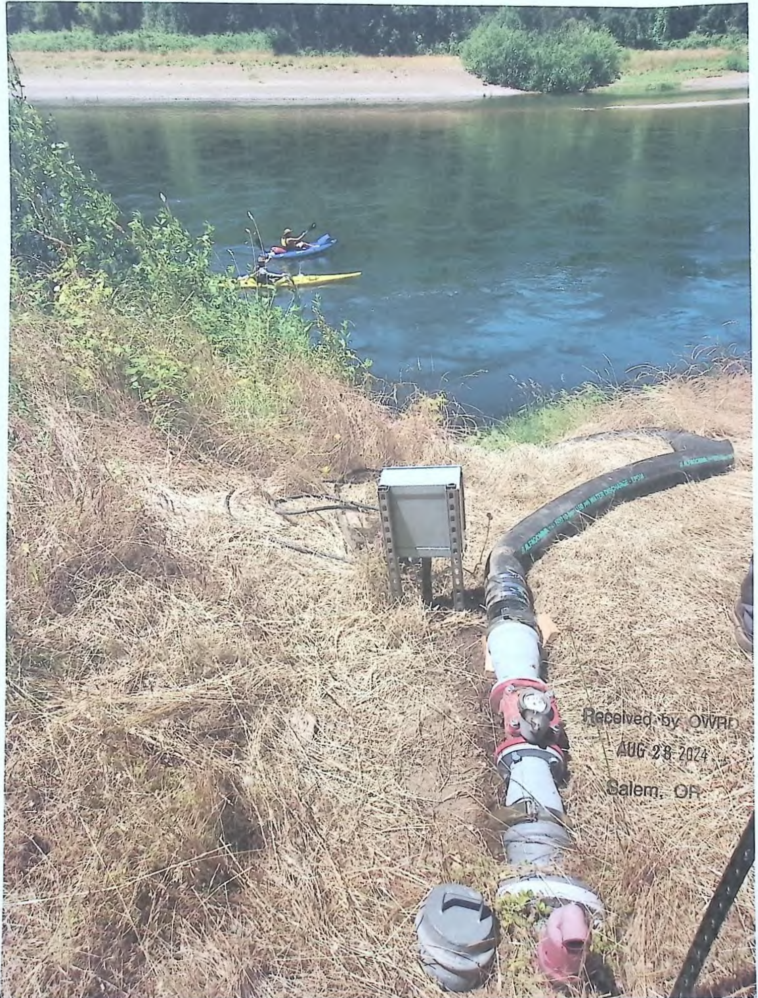
6-24-24 WEM Green Gold Ag COBU 10 HP River Pump Flow Meter Location
