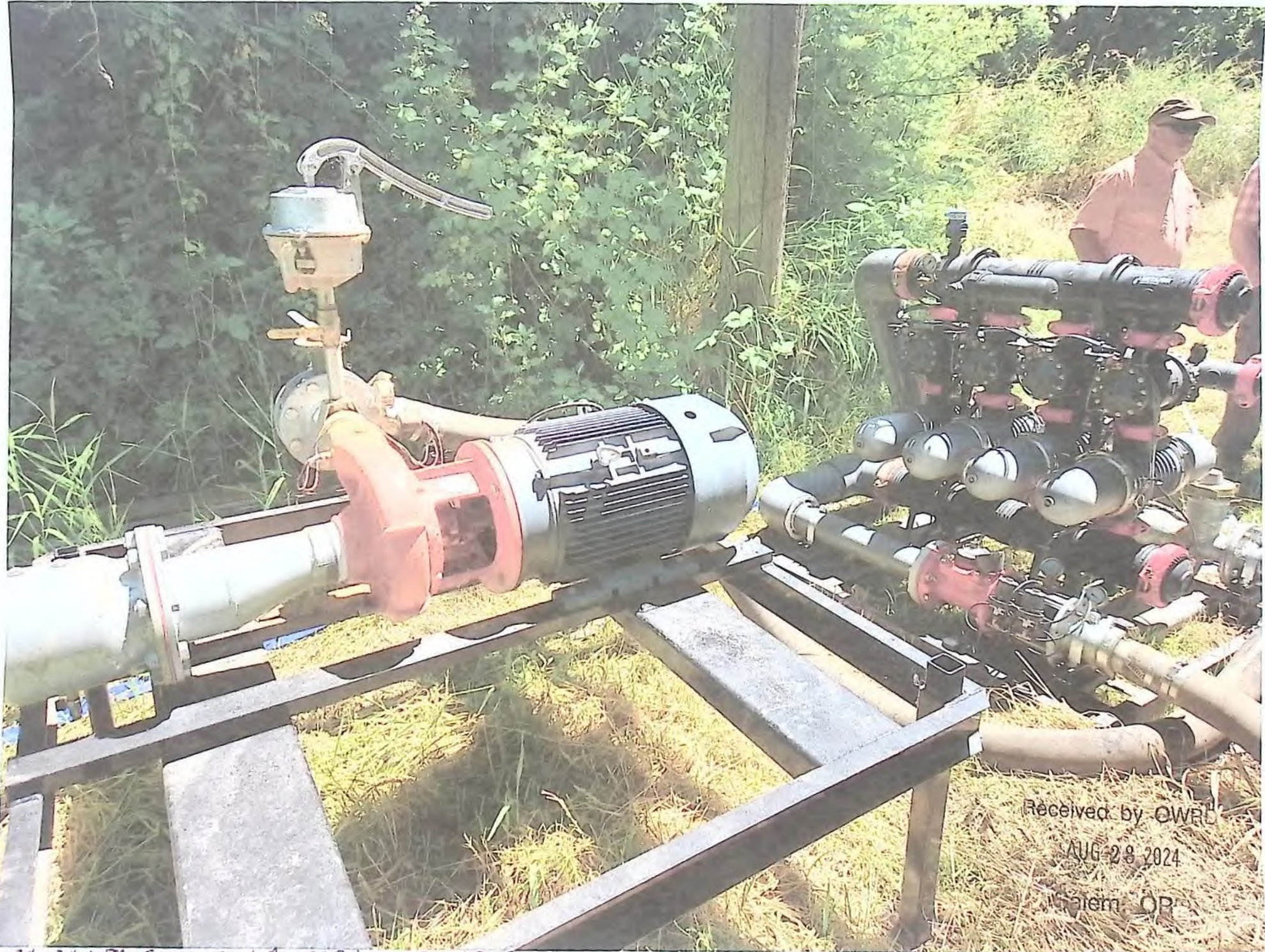
G-24-24 WMA Green Gold Ag CDBU 30 HP Bulge Pump Flow Meter Location
