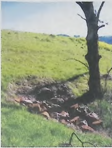
Thursday, April 04, 2002 Westbrook - 9s3w14 Ra-84703 Outlet area for overflow pipe.
