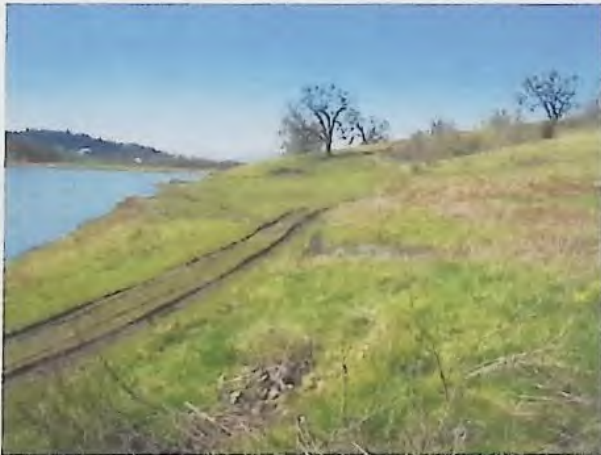
Thursday, April 04, 2002 Westbrook - 9s3w14 Ra-84703 Emergency spillway located on north end of dam. Spring area along north shore u.s. from emergency spillway.
