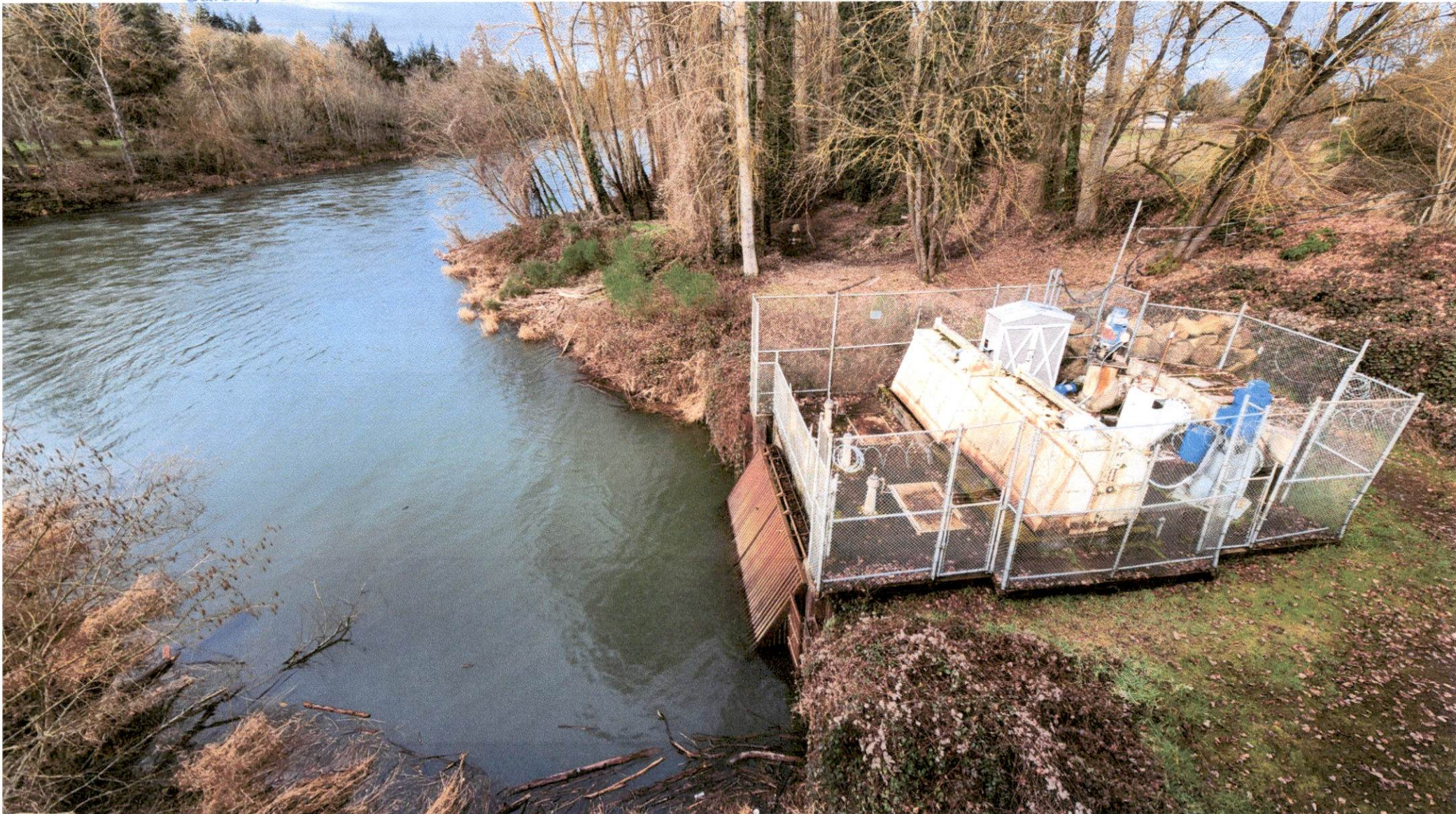
Perrott COBU Site Inspection 2-20-2025 Muddy Creeks Irrigation Project POD 1
