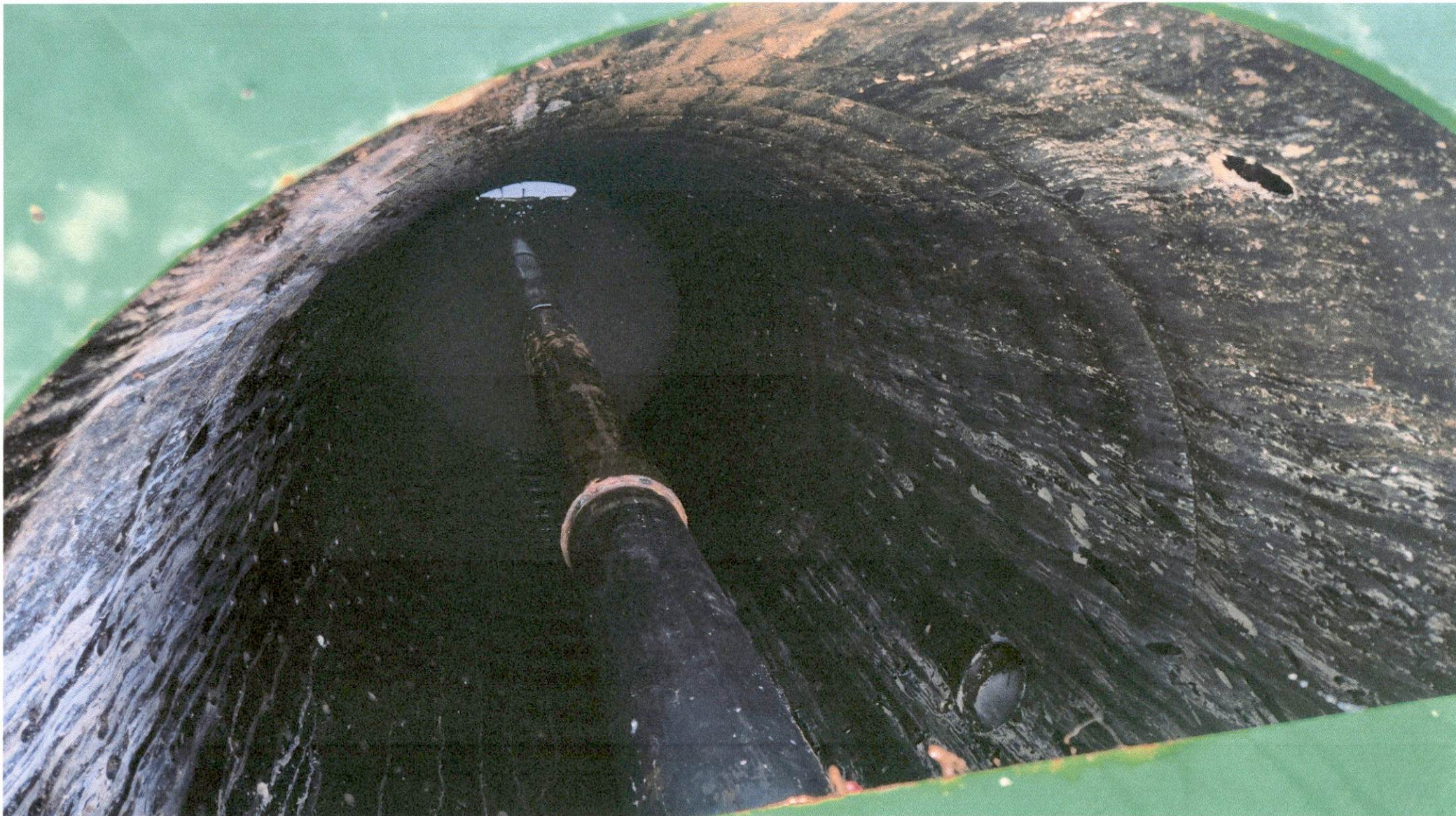
Perrott COBU Site Inspection 2-20-2025
