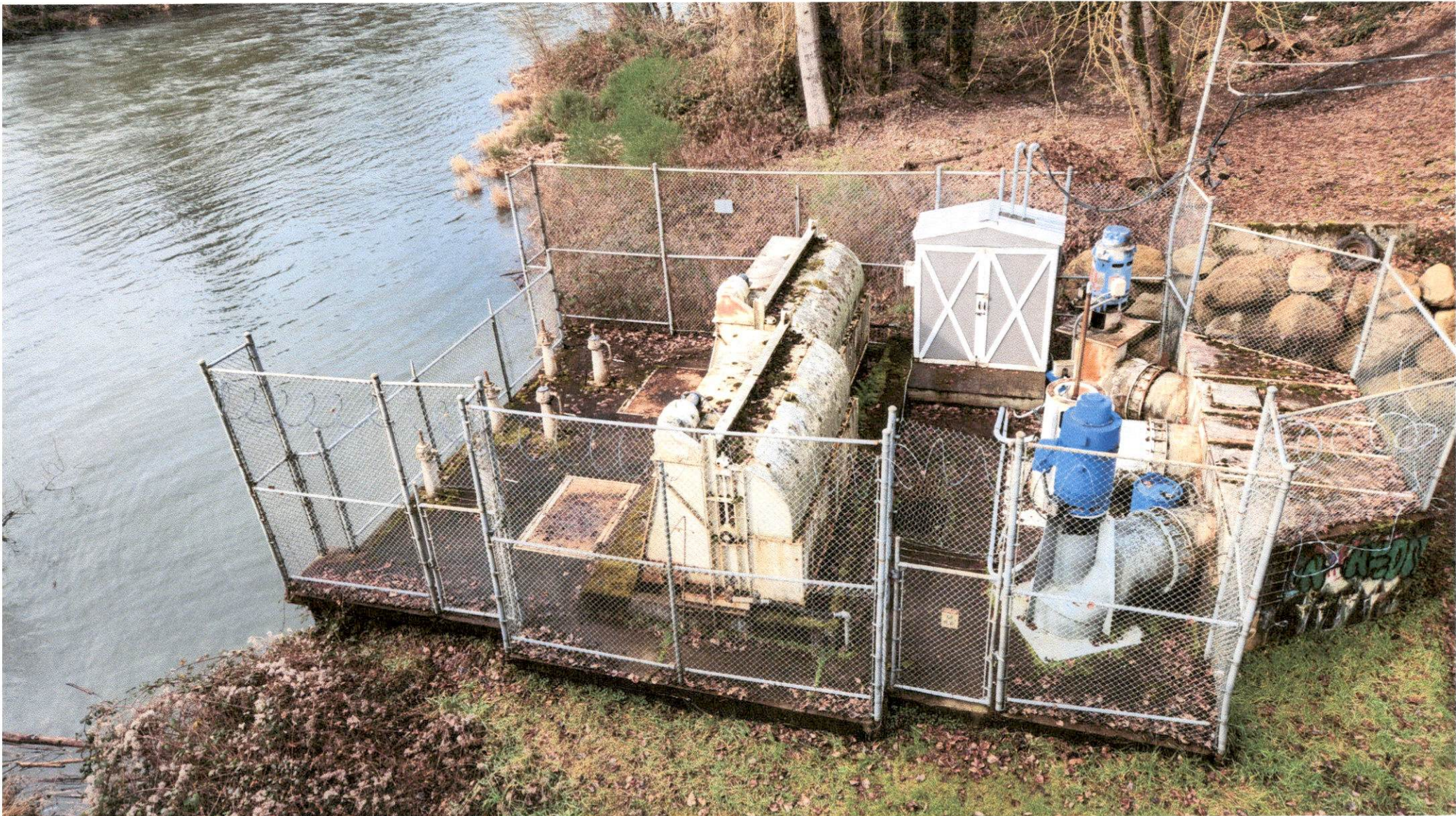
Perrott COBD Site Inspection 2-20-2025
