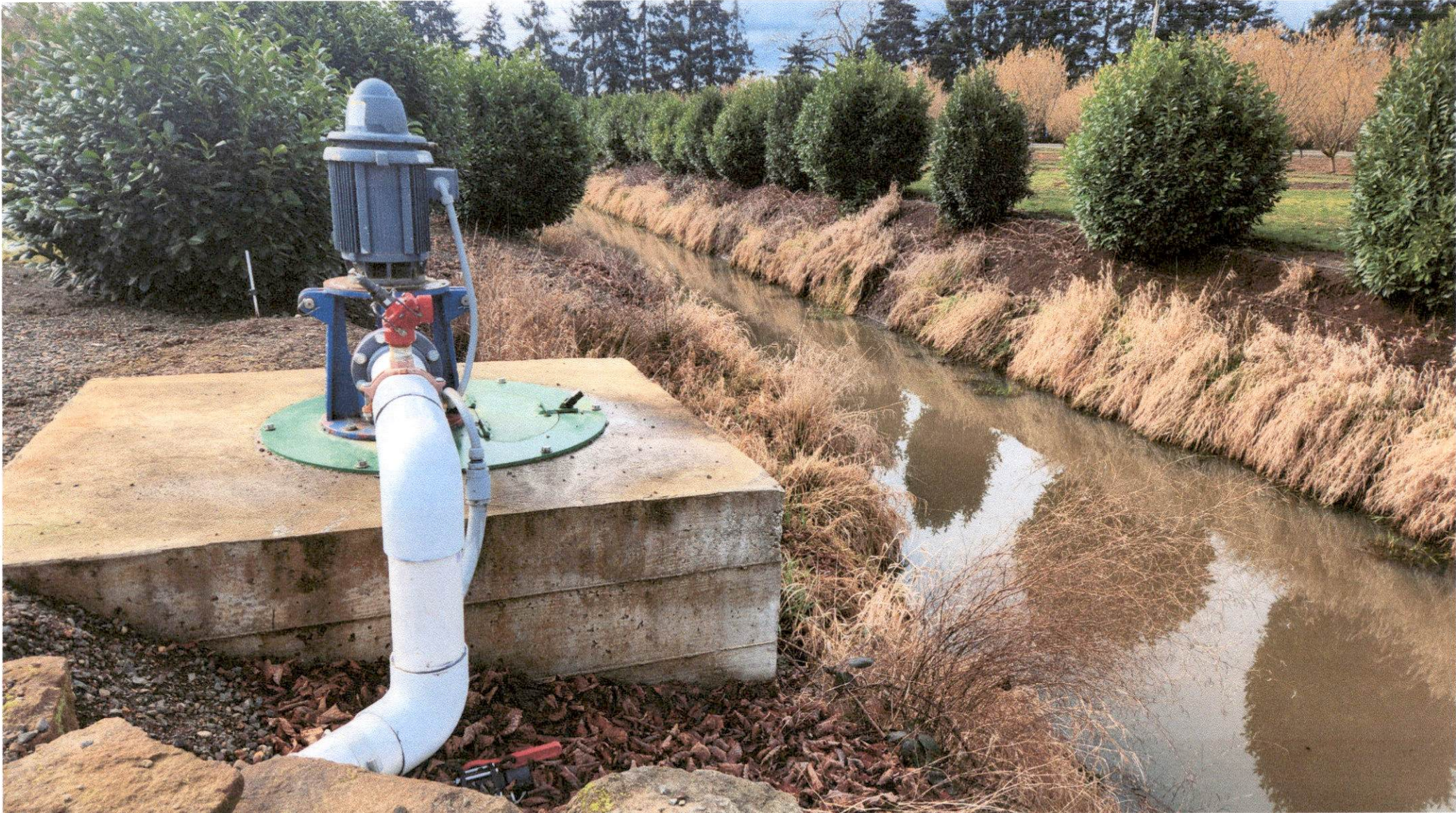
Perrott COBU Site Inspection 2-20-2025 Perrott Re-Diversion POD Pump and Sump Site
