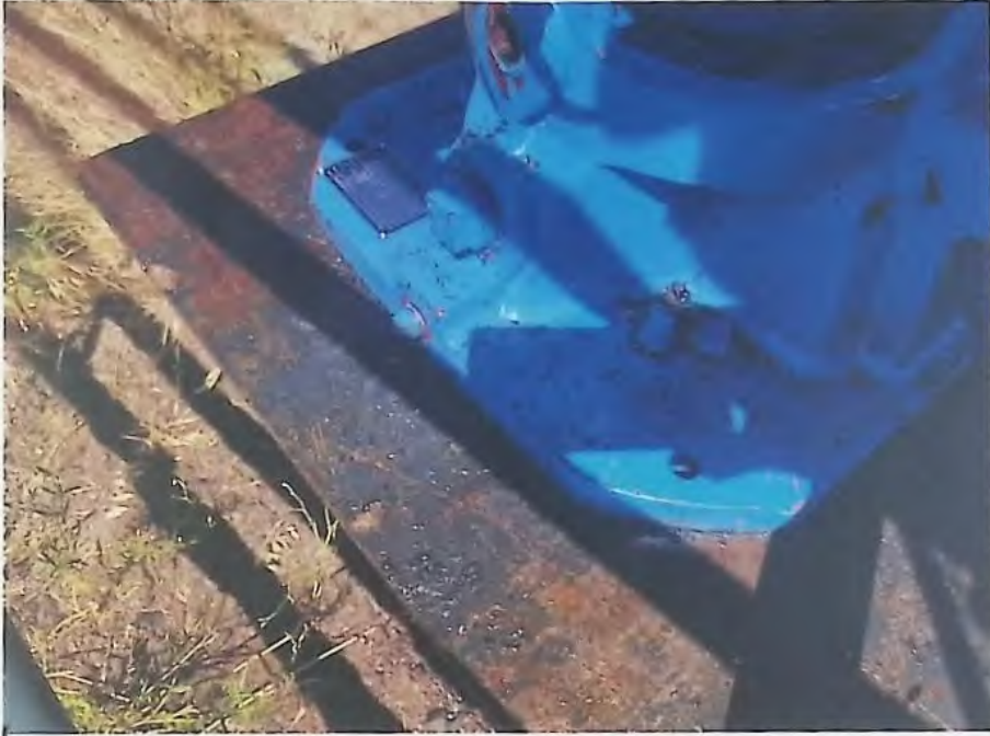
Well #5 Access Port
