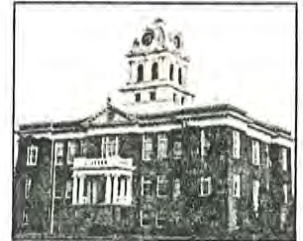
CROOK COUNTY COURTHOUSE PRINEVILLE, OREGON 97754
