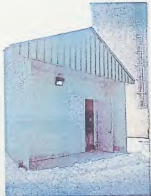
Photo 8: Well No. 1 Building
