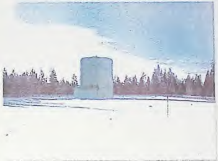
Photo 6: 1.2 MG Reservoir and Well No. 1
