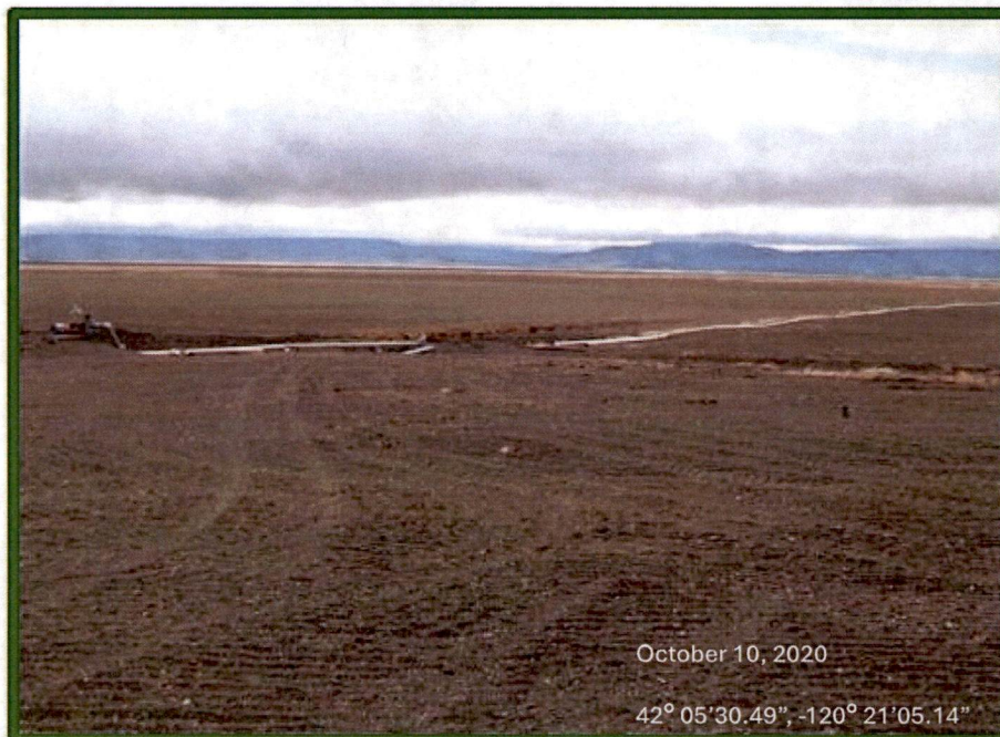
Figure 5. 3,600 feet of 8" mainline, looking southwest.
