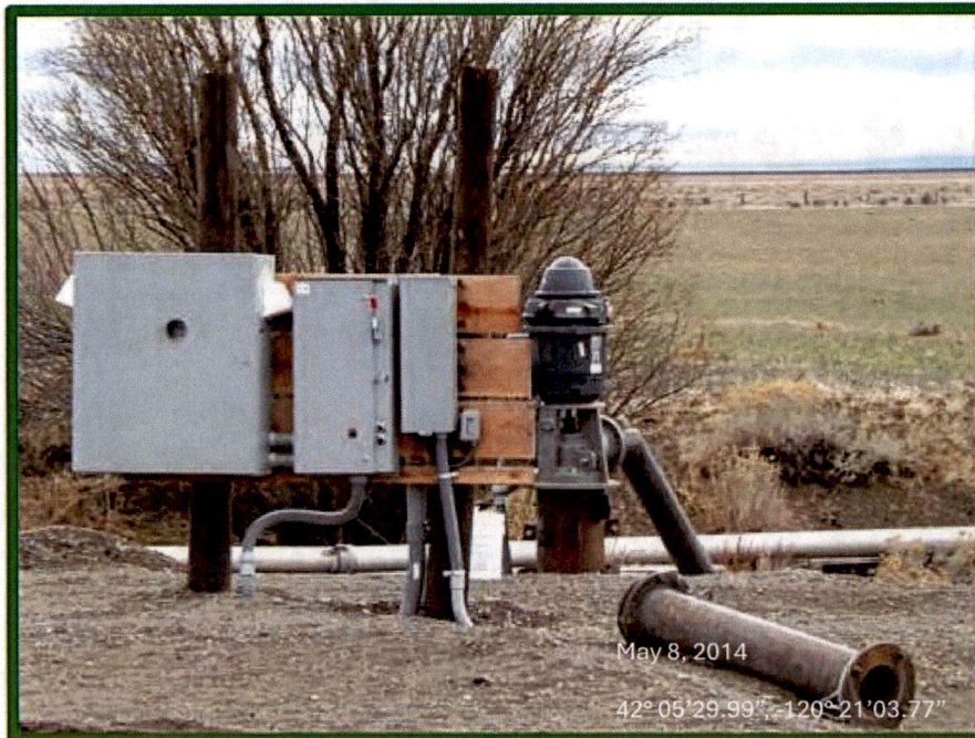
Figure 4. 40 HP Turbine Pump and Electric Panels. Looking south.
