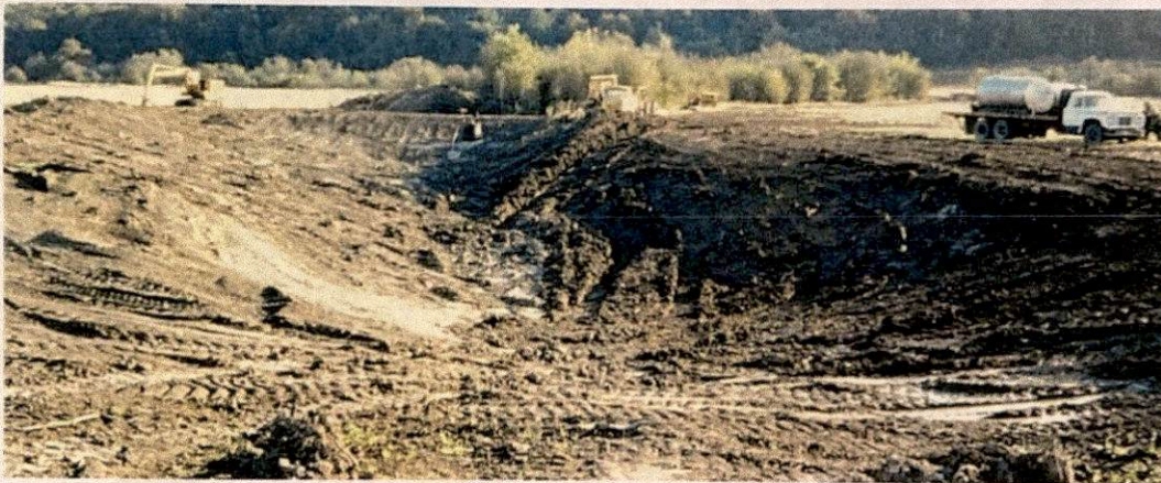
CREATING THE RESERVOIR & MOVING THE EARTH
