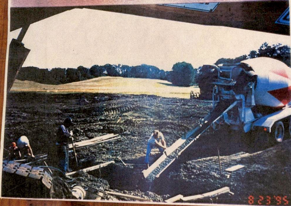
CONSTRUCTION OF "PANDA" 1995
