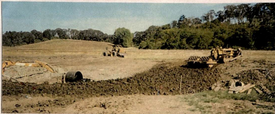
COMPACTING THE DAM FOR POND "A"
