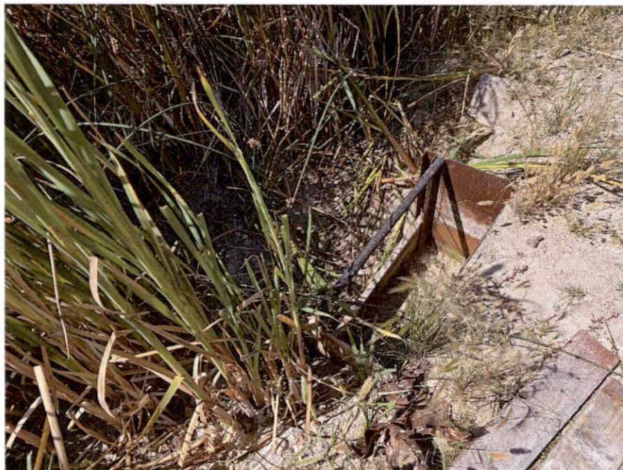
Headgate in Earthen Structure for Distribution
