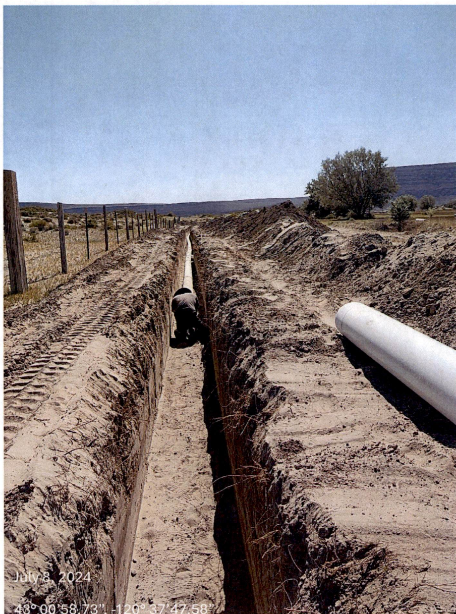
Figure 19. Installing 10" PVC underground pipeline – looking east. Total length of pipeline = 3,600 feet.
