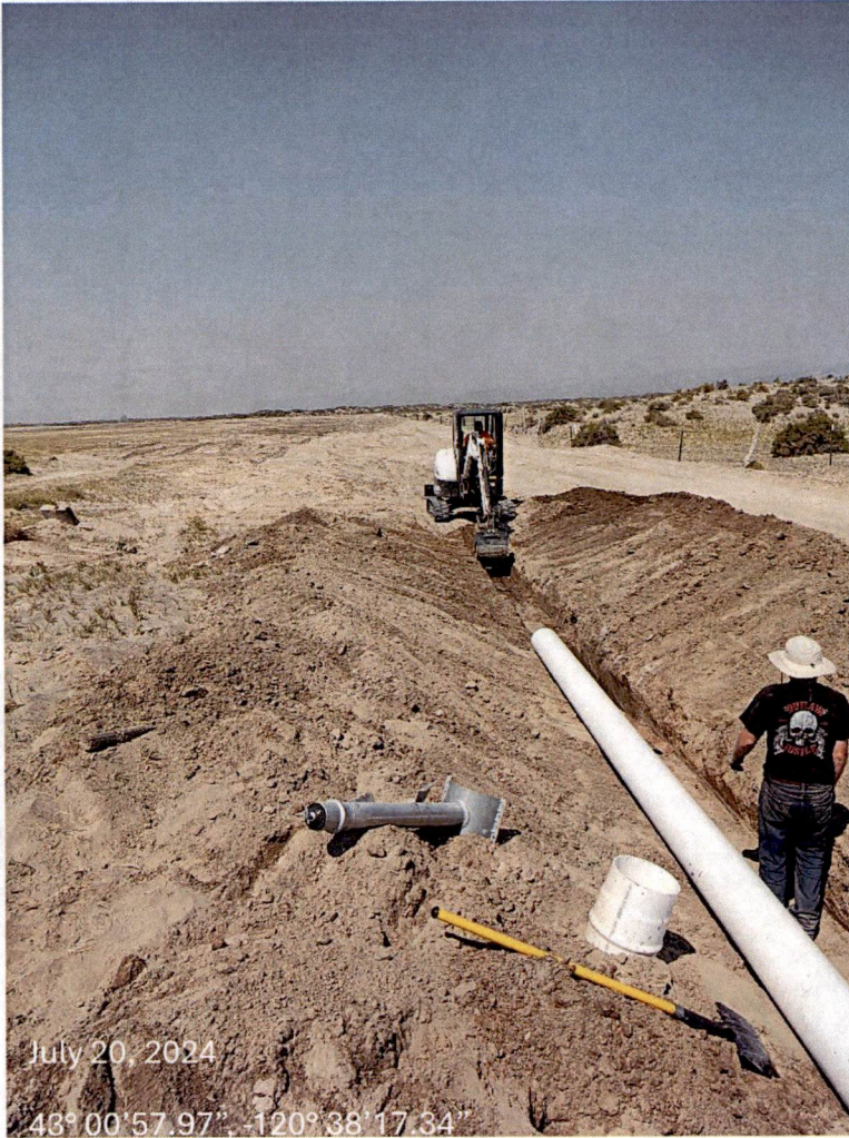
Figure 23. Installing 10" underground PVC Pipeline with excavator near the start of Levee #1. End of Pipeline #1. Looking west.
