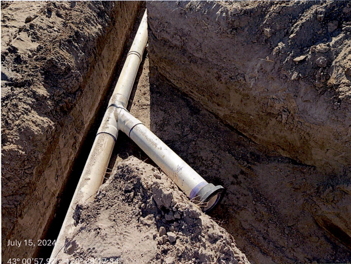
Figure 22. Installing 10" underground PVC Pipeline and Stubouts (1 of 15) with 10" butterfly valves.
