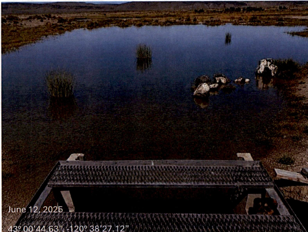
Figure 2. On natural levee, looking northeast towards Well #1. Water flowing through concrete headgate with catwalk.
