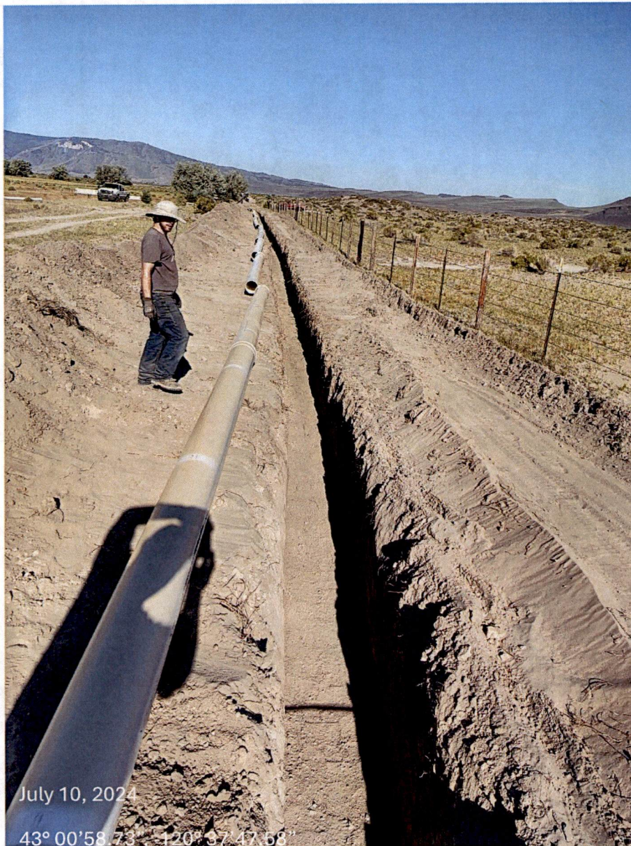
Figure 21. Installing 10" underground PVC Pipeline – Looking west.
