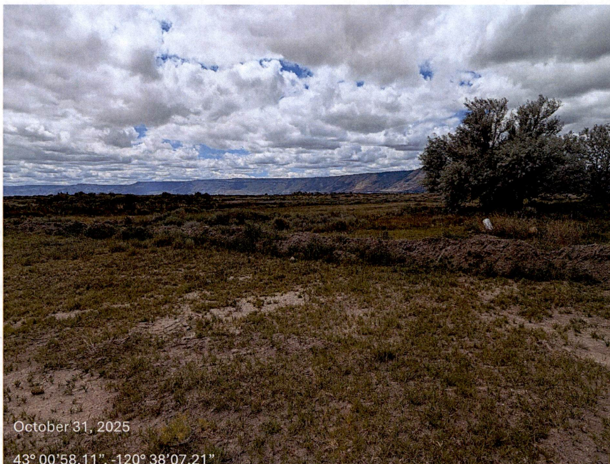
Figure 16. Buried 4" PVC Pipeline connecting Well 1 to 10" PVC pipeline from Well 3.
