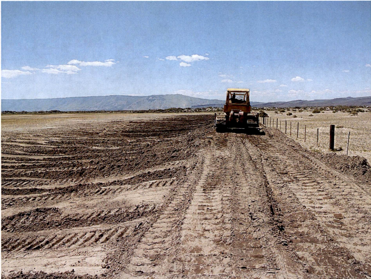
Figure 4. Building Levee #1 (1 of 3 Levees) with D7 Dozer on July 15, 2024. Levees are 12 foot wide on top with a 3 to 1 slope). Levee #1 = 2,000 feet in length, Natural Levee = 2,002 feet, Levee #3 = 1,700 feet.
