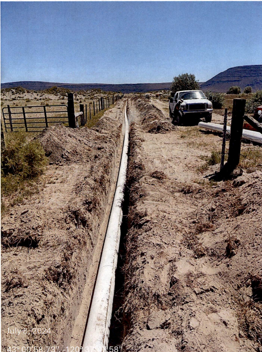
Figure 20. Installing 10" underground PVC pipeline – Looking east.
