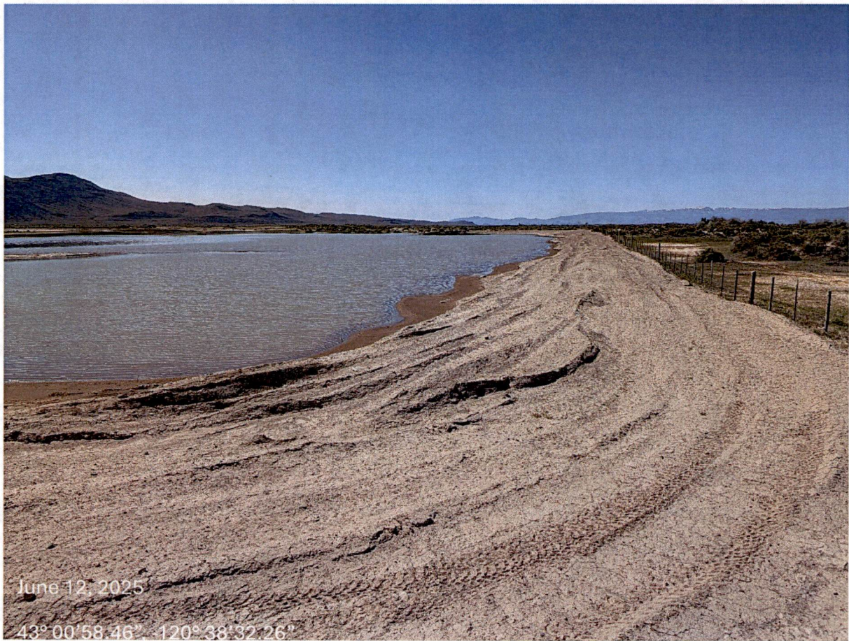
Figure 5. Levee #1 - Looking South – Raising water level to flood south end of property.
