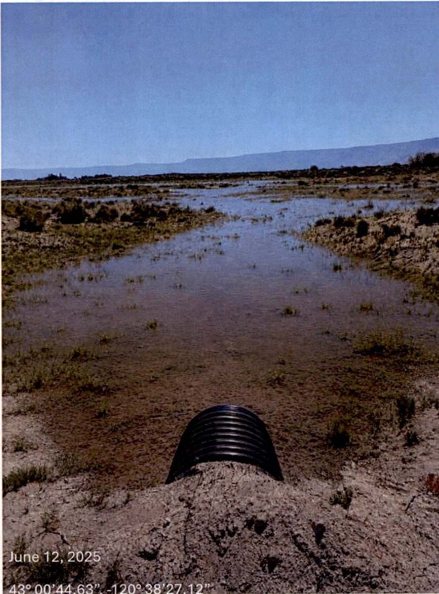
Figure 3. On natural levee looking southwest. Outlet of culvert.
