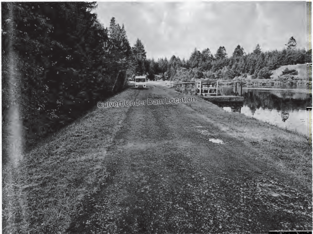
Figure 10. Simpson Creek "Amos" reservoir dam, with denotation of culvert moving water from fishway under dam.
