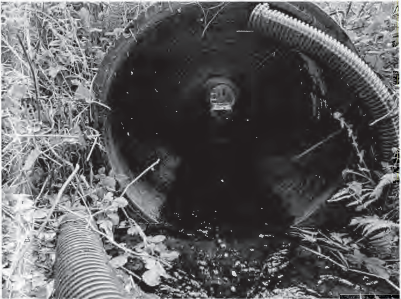
Figure 12. Simpson Creek "Amos" reservoir water conveyance culvert under the dam. Image is view looking upstream from downstream end.
