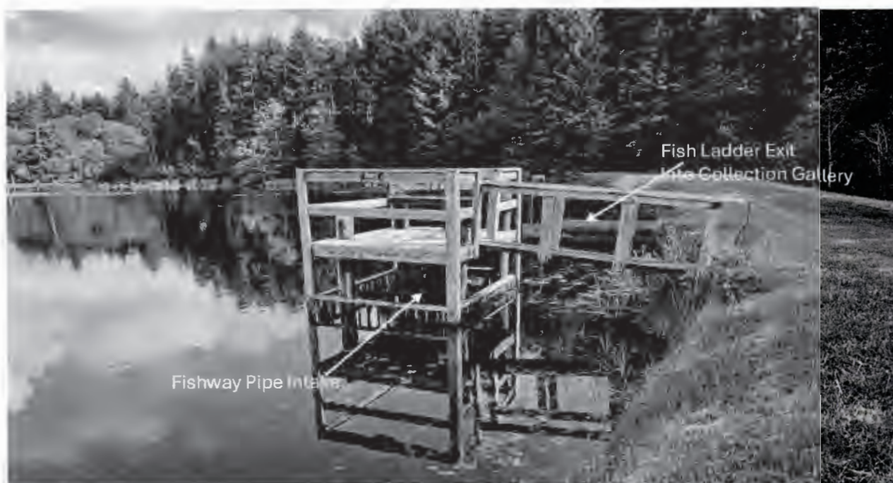
Figure 3. Simpson "Amos" reservoir fishway intake. Data collected ODFW 05/12/25.
