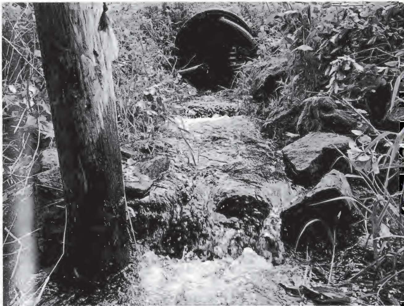
Figure 11. Simpson Creek "Amos" reservoir dam, with denotation of culvert moving water from fishway under dam.
