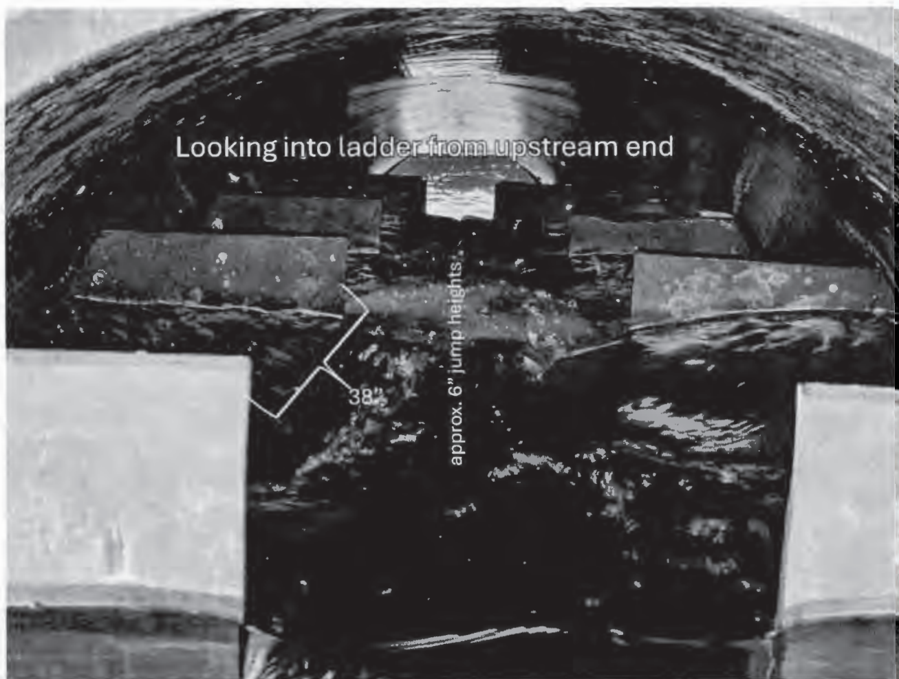
Figure 5. Simpson Creek "Amos" reservoir fishway. Imaging looking into fishway from upstream intake. Data collected ODFW 05/12/25.
