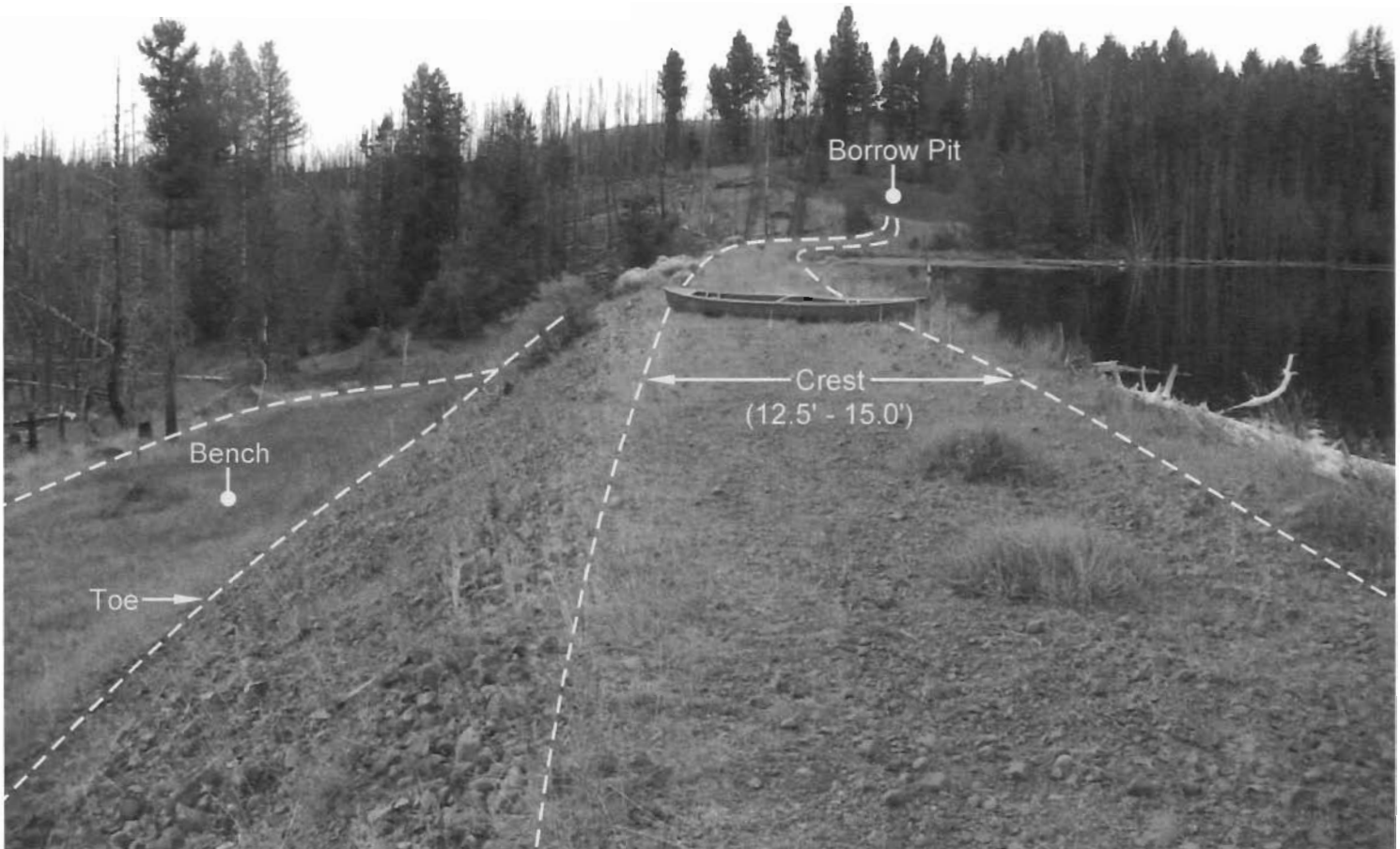
Figure 6 Dam Crest View to South
