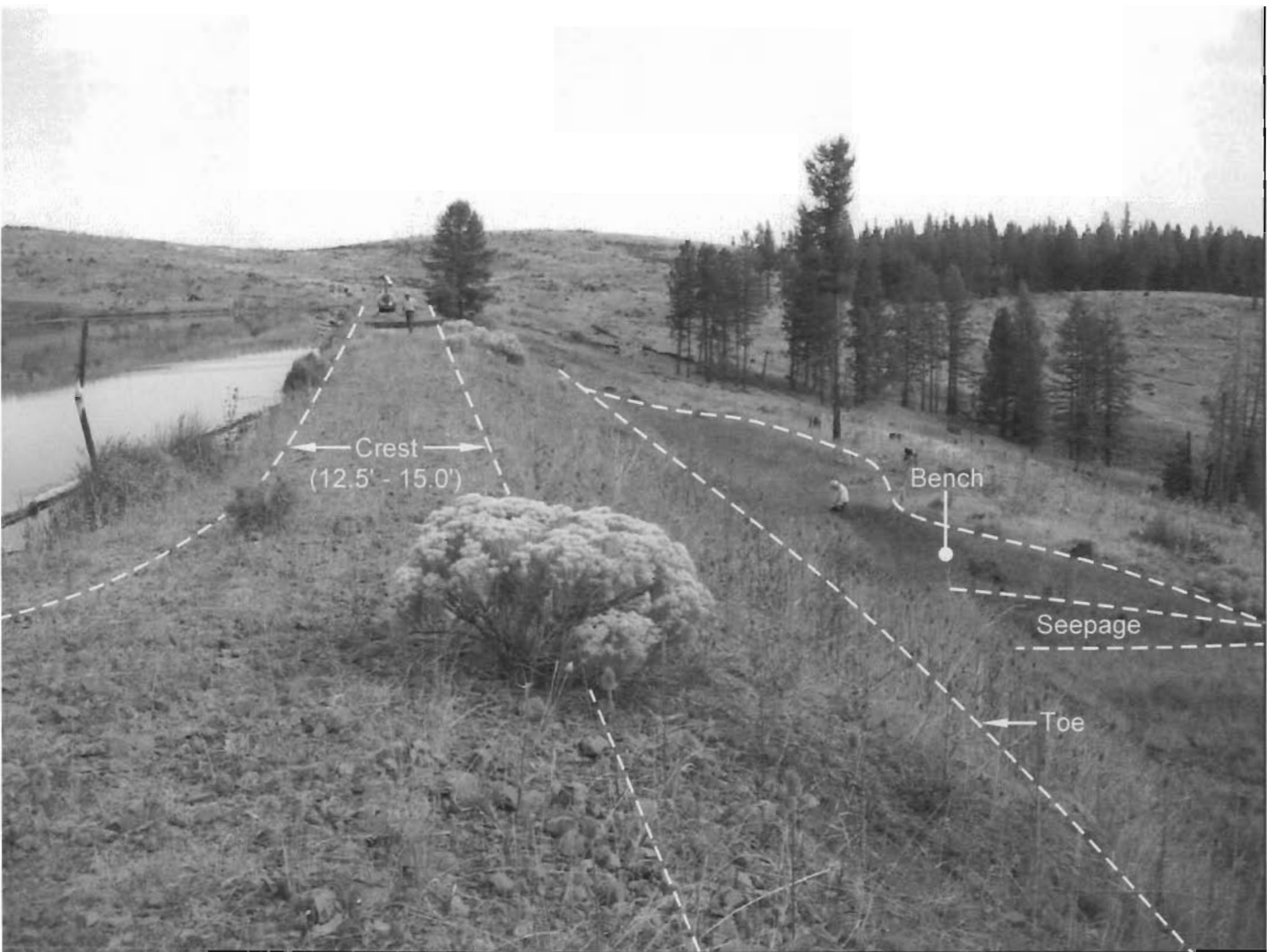
Figure 7 Dam Crest View to North
