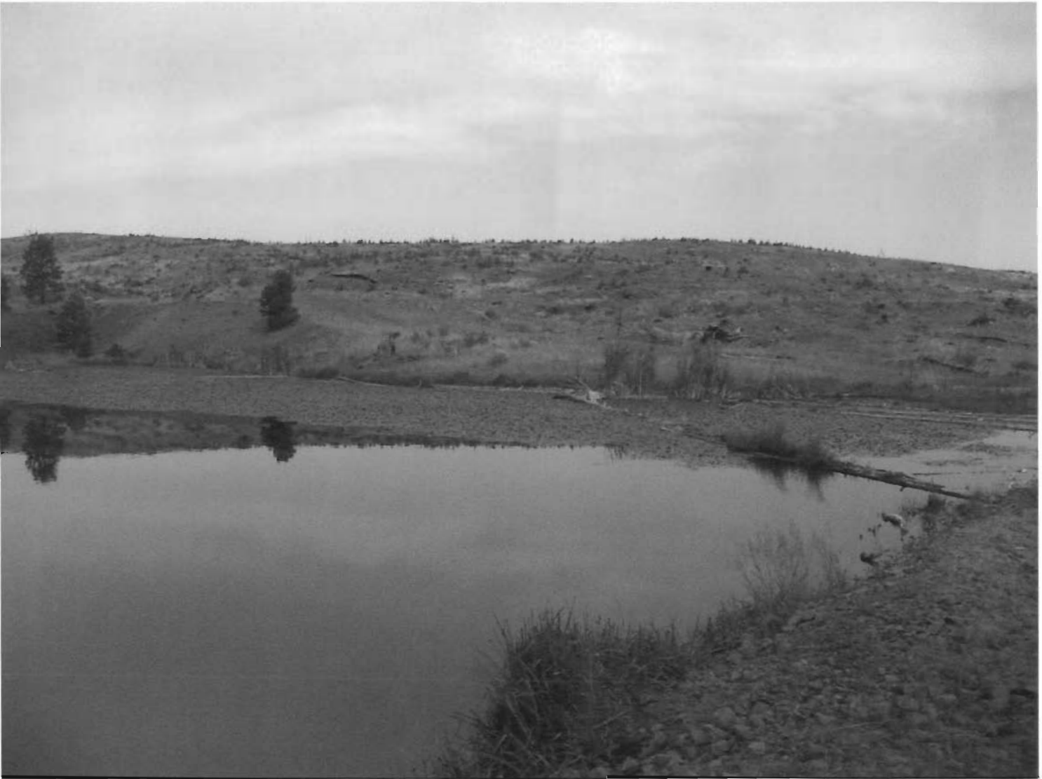
Figure 10 Inlet to Emergency Spillway View to North North-West
