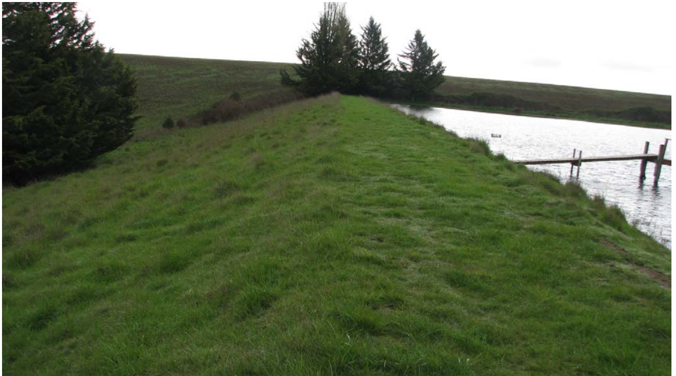
Figure 1. Upstream and downstream slopes and crest of dam showing the excellent control of woody vegetation on the dam.
