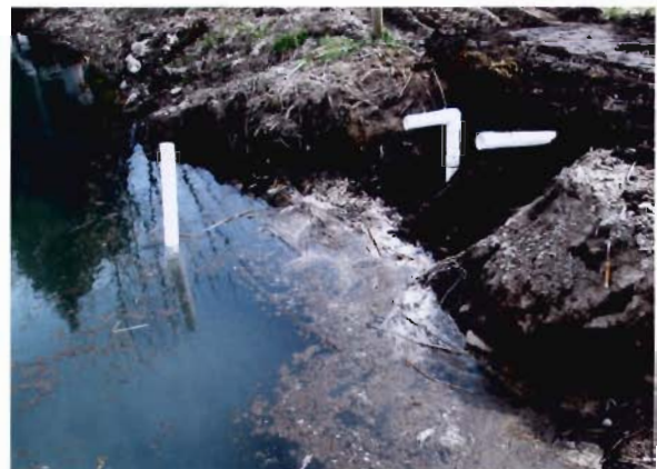
Pond partially filled before adjusting outlet pipe length (height) to establish water level
