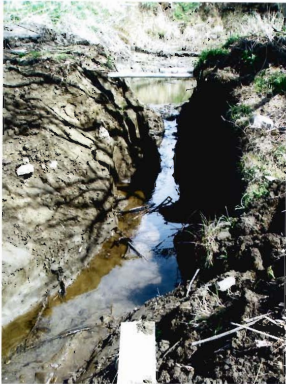
Prior to placing outlet pipe
