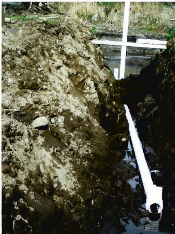
Outlet pip in place
