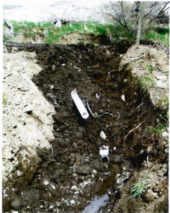
Backfill over outlet pipes
