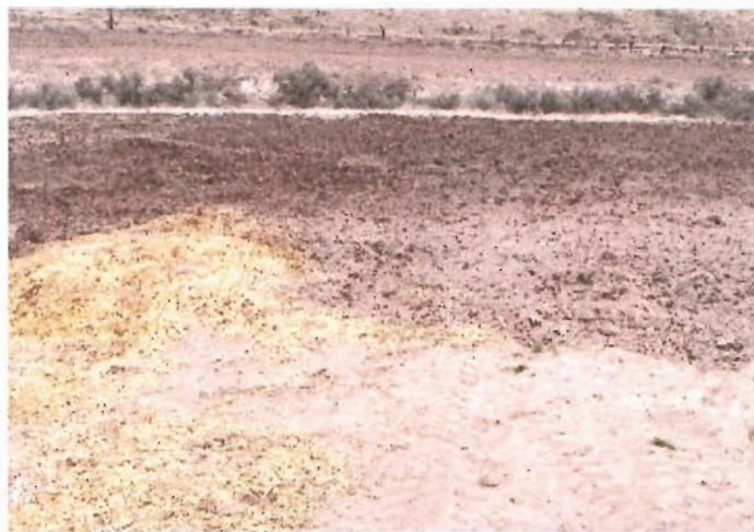
#4 Emergency Spillway from the lowest point in the reservoir
