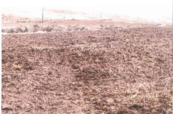
#5 Emergency Spillway topography looking NW
