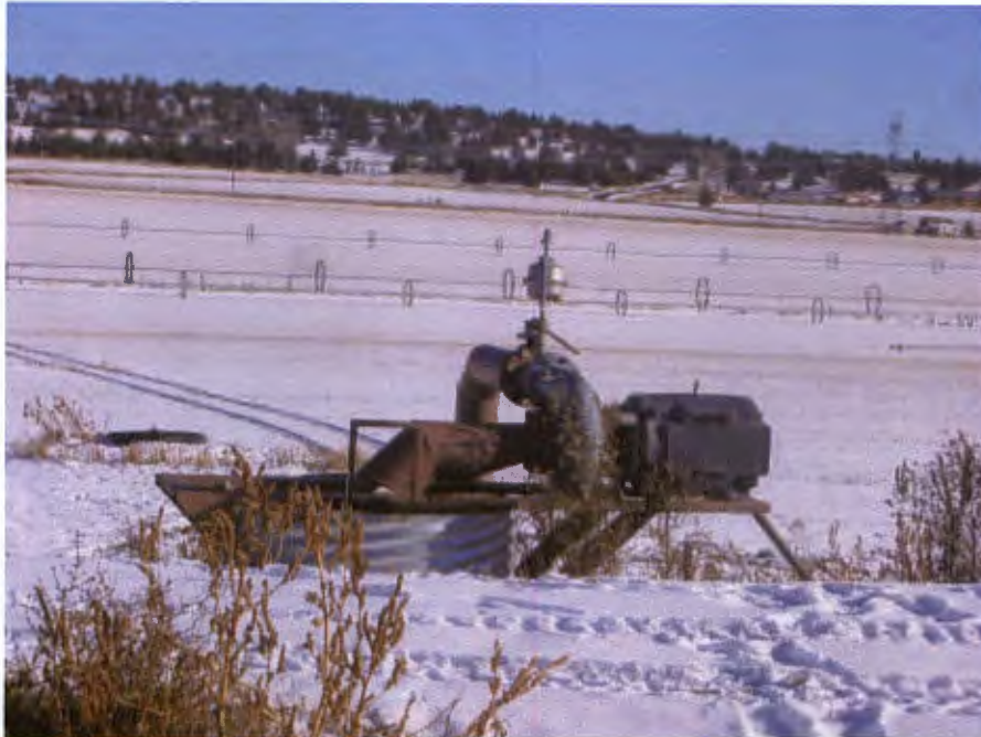
PRIMARY IRRIGATION PUMP FROM CANAL
