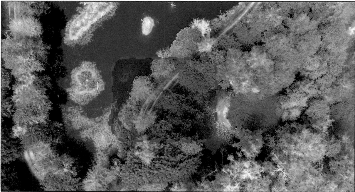
Figure 4-1. The spillway location between pond and Five Rivers at the southeast corner of the pond. Water drains through an existing 24" diameter pipe from the pond towards Five Rivers.
