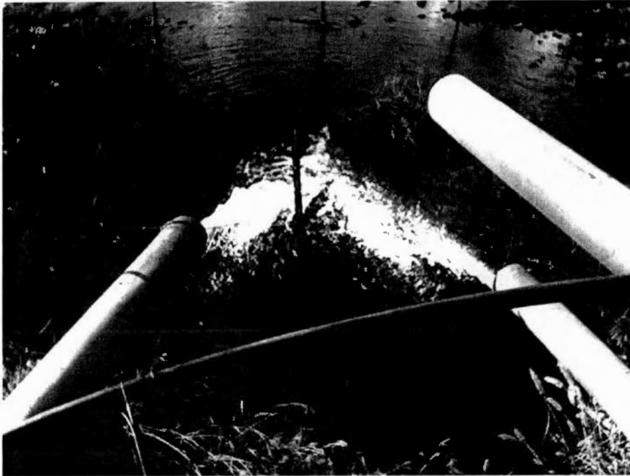
DISCHARGE INTO IRRIGATION CANAL
