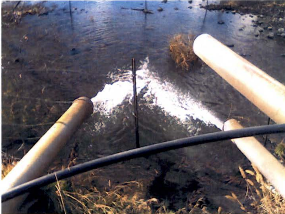
DISCHARGE INTO IRRIGATION CANAL
