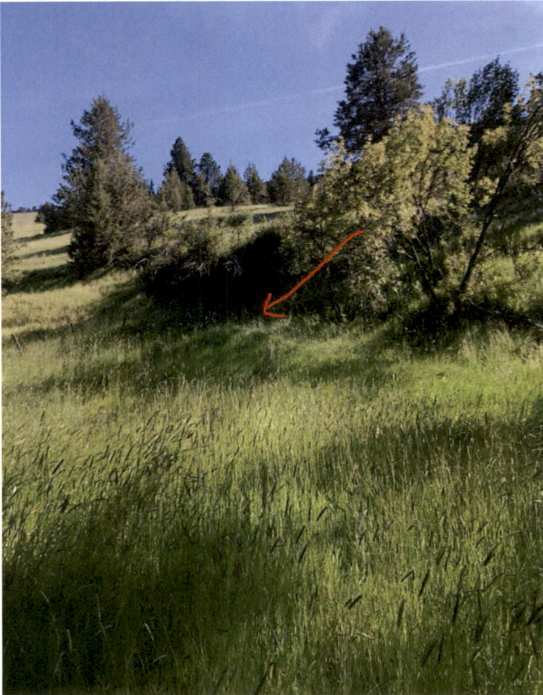
EMBANKMENT FROM DISTANCE
