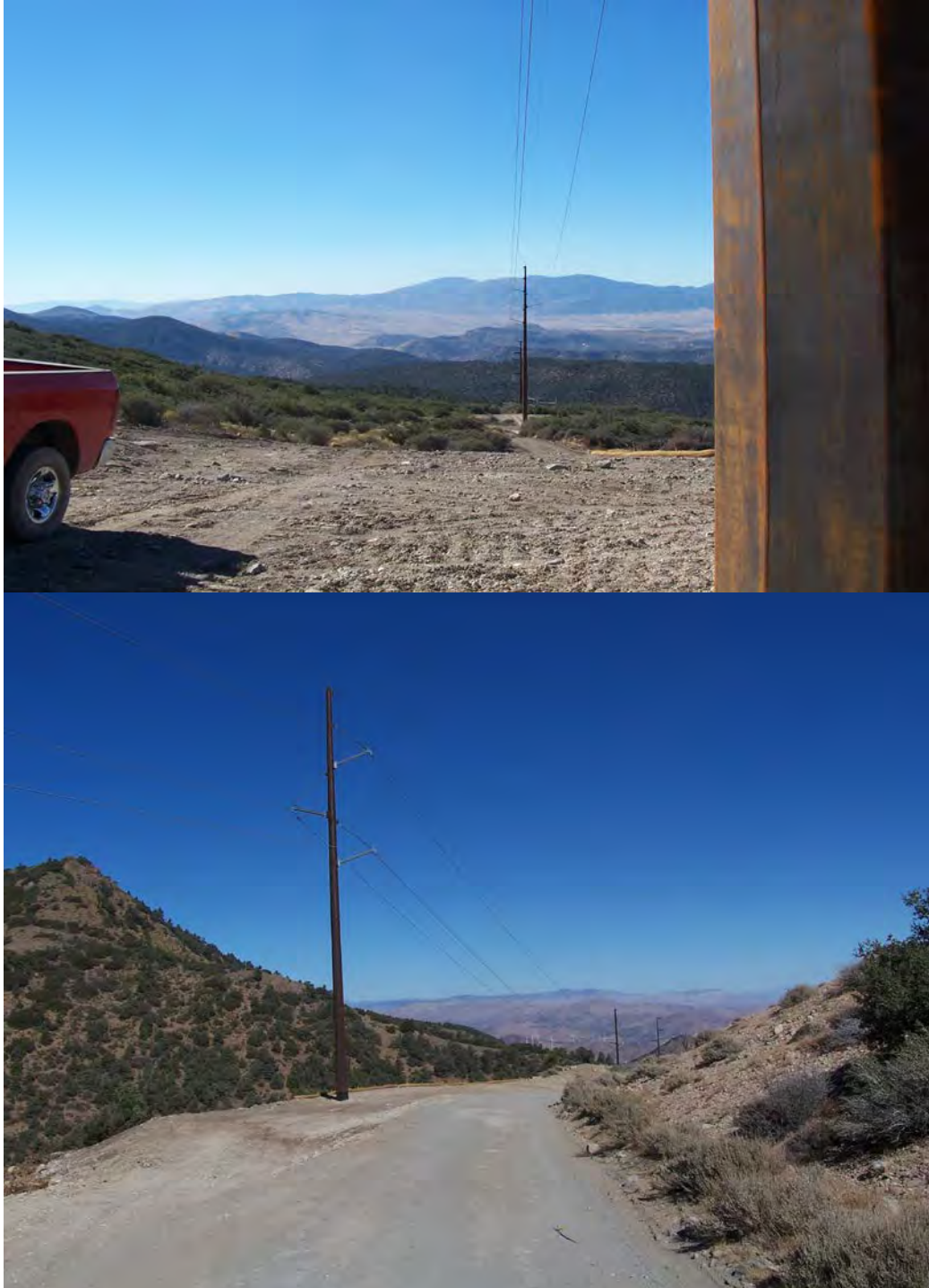
Figure 3-19. Photograph of an existing single circuit steel mono-pole transmission line similar to the one proposed for the Swan Lake North Hydroelectric Project (Source: Electrical Consultants Inc. 2019)
