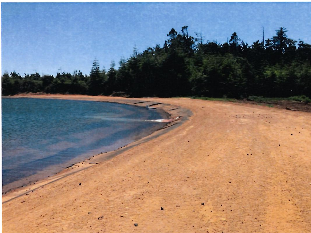
Lake Tony – View of pond liner and wide maintenance road
