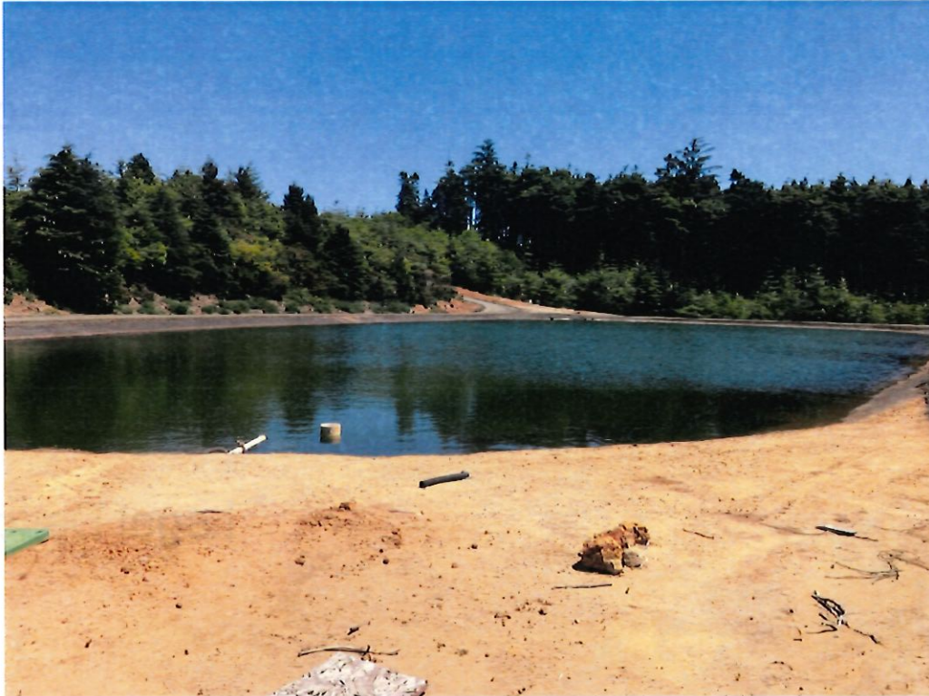
Lake Tony – View of pond, liner and inlet pipe. Looking southeast.
