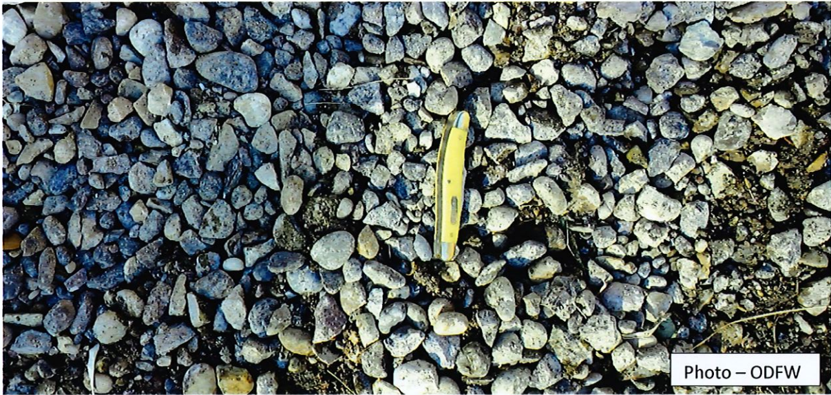
Figure 3. Gravel covering pipe with 4" pocket knife for scale.
