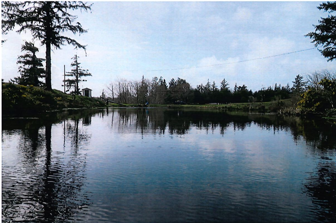
Reservoir #1 facing downstream.
