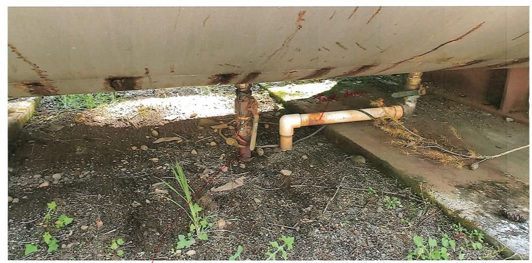
RECEIVED JUN 21 2021 OWRD 5/u/2021 COBU Eagle fer Camp - outlet from tank to 1R/CM system, gravity flow 2" galvaized pipe
