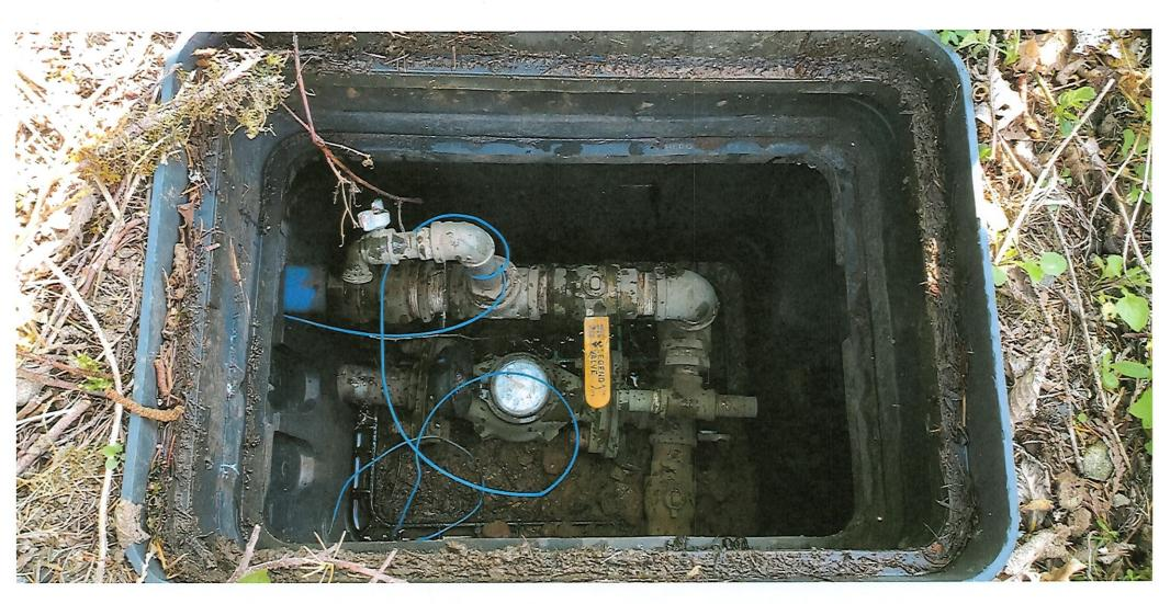
RECEIVED JUN 2 1 2021 OWRD 5/11/2021 COBU Engle Fern Comp Flow Meter / Well discharge 2" Q.D. galvanized pipe (Hersey)
