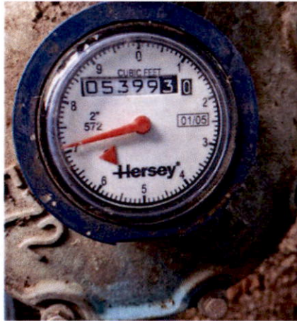
2. Flowmeter after 1.5 minutes of pumping
