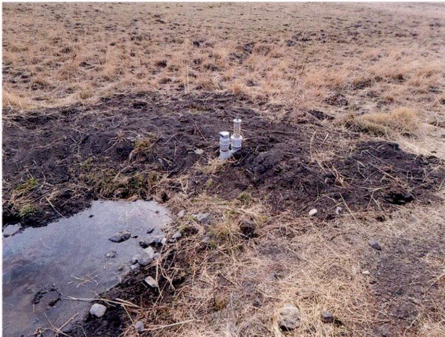
Well #1 Flooding Mainline
