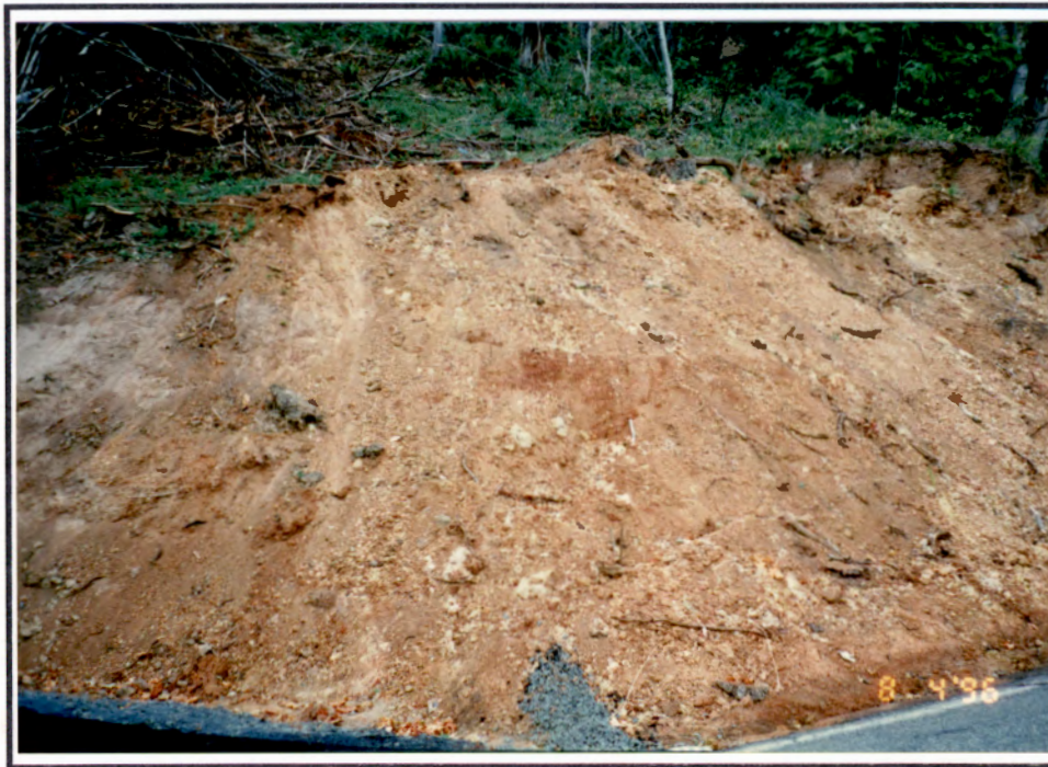
Photo 4. Road cut showing sandstone and siltstone horizons. Red color of rock is due to iron rich minerals, possibly the cause of high iron groundwater in the vicinity.
