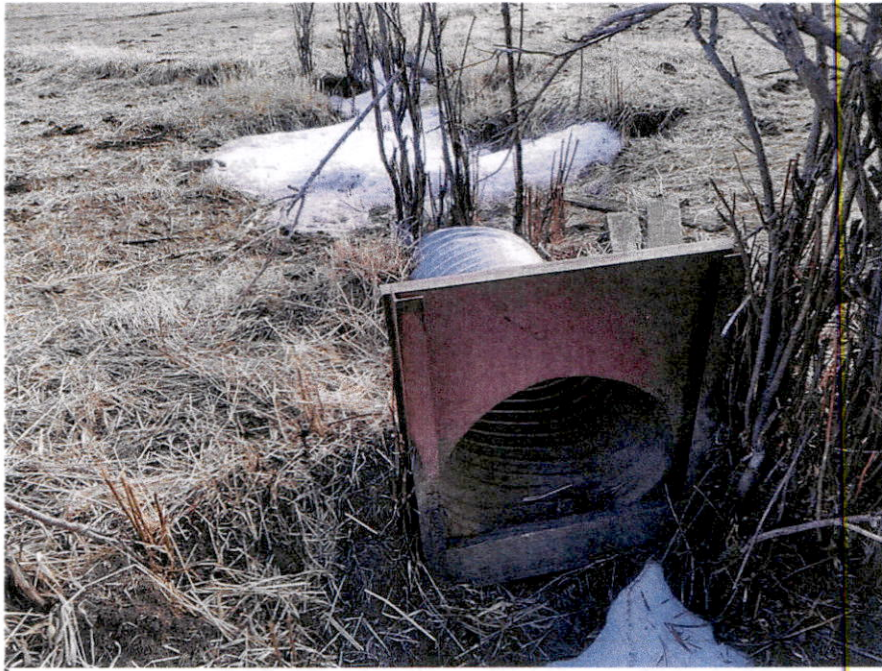
Typical Headgate for Flooding
