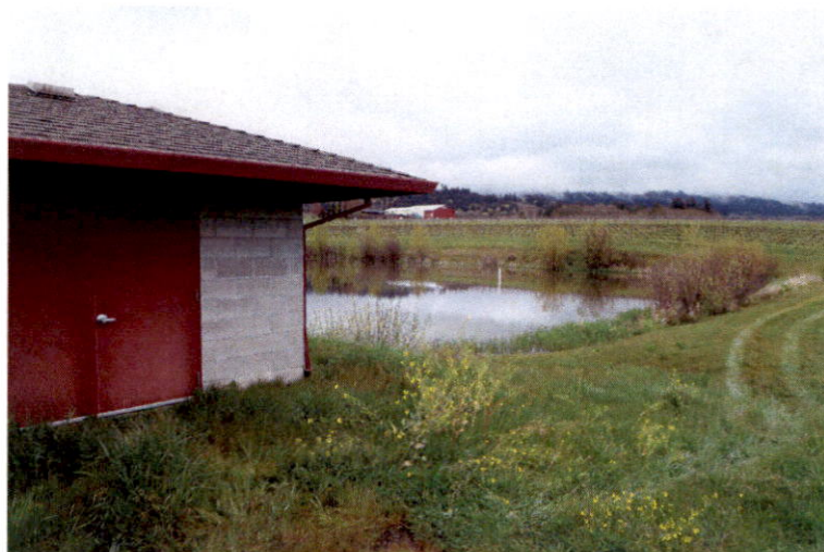
Pump house by pond.
