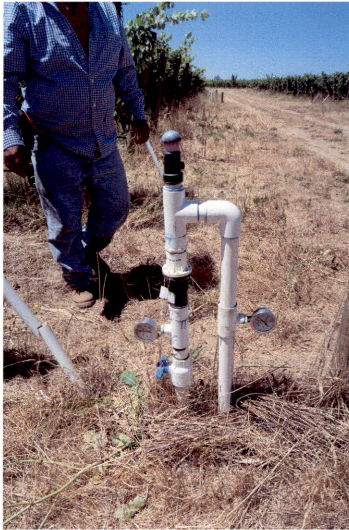
Zone plumbing with pressure reducer and pressure gages, typical.
