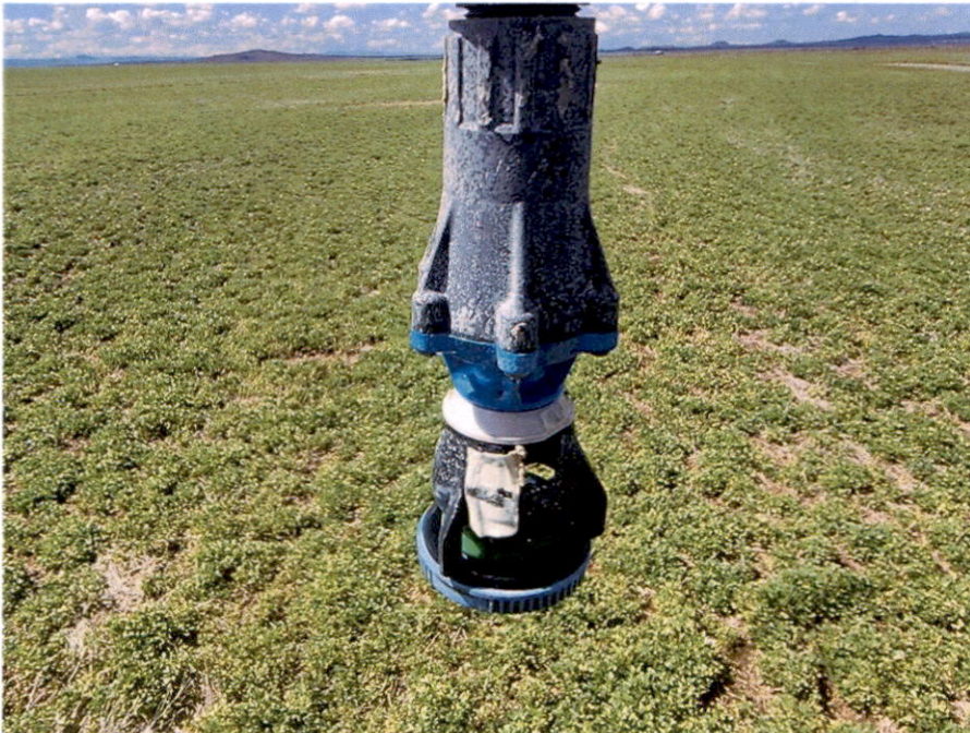
Well #8 Typical Nozzle
