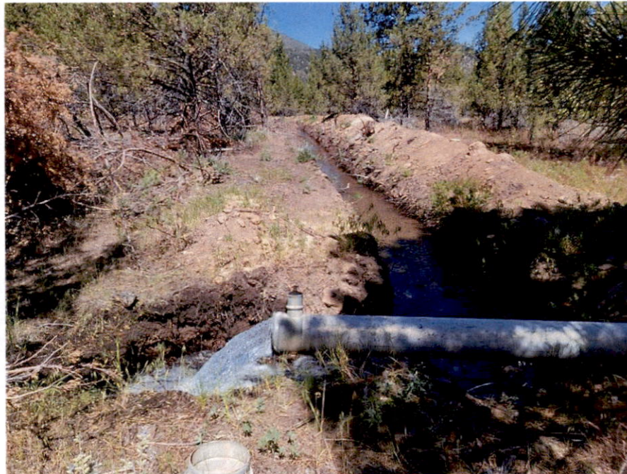
Pump Discharge at Ditch
