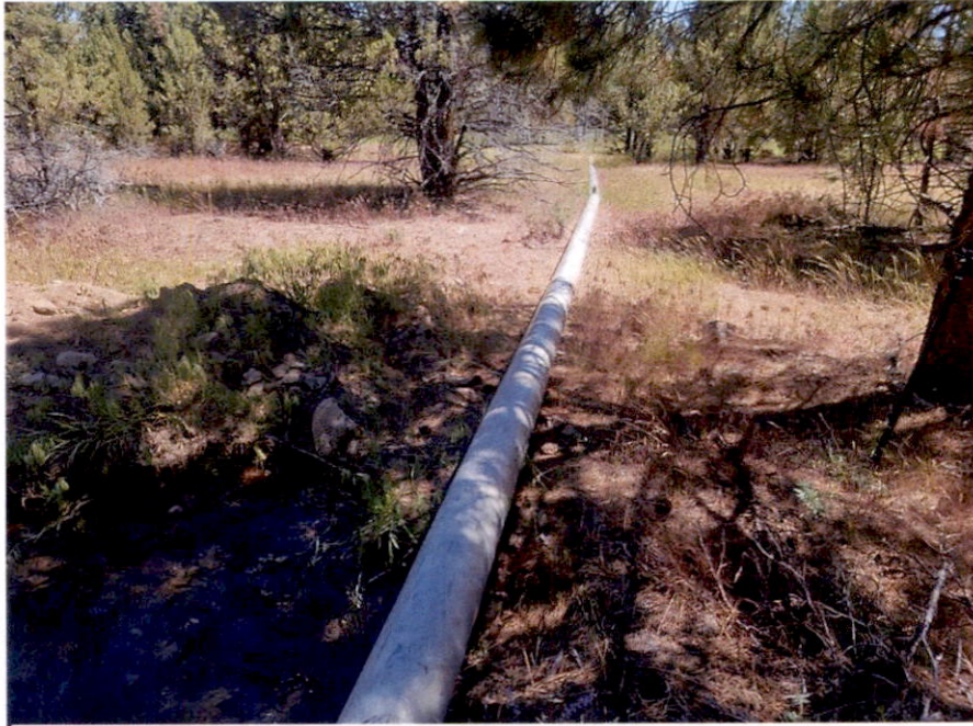
Piping from Well to Ditch
