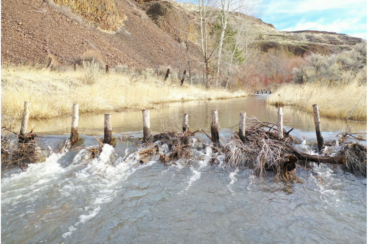
Thirtymile Creek with a beaver dam analog - a key implementation strategy for the creek (Herb Winters photo credit)
