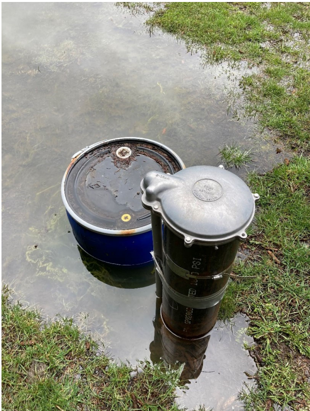
Well inspection in the NC Region
