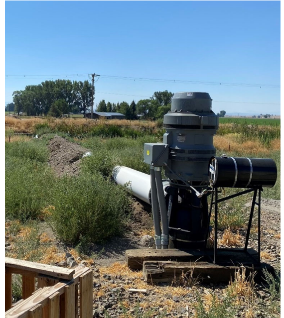
Large diameter well, SC Region
