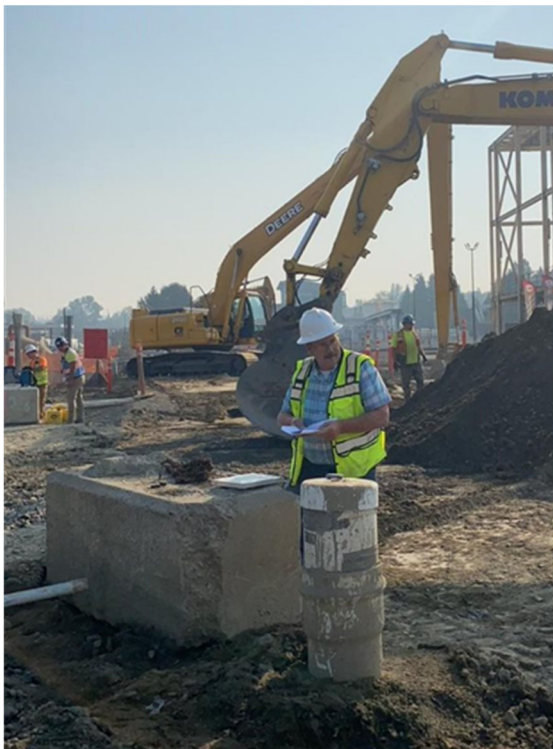
Inspecting a temporary dewatering well
