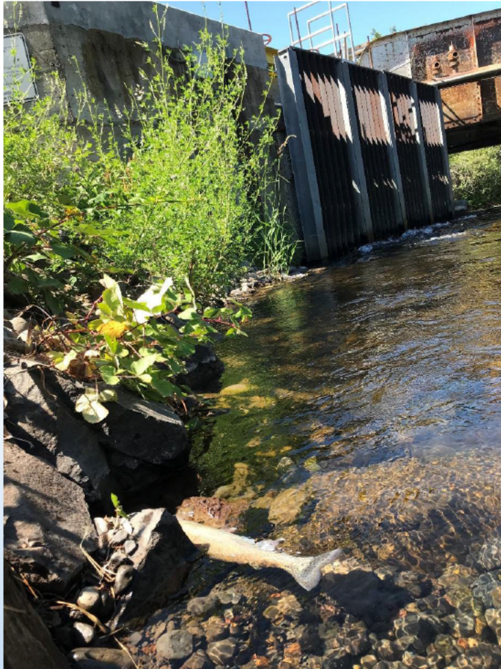
Dead Mid-Columbia steelhead at Walla Walla River diversion.
