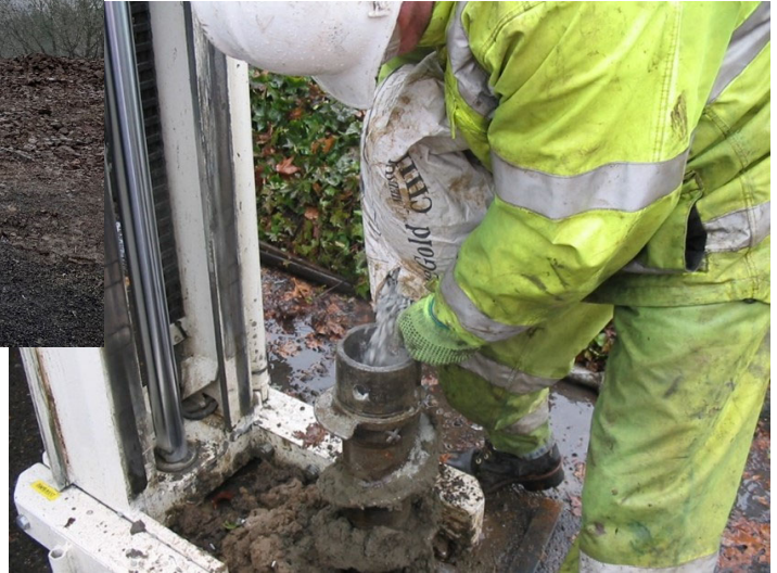
Abandoning a monitoring well
