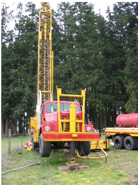
New well under construction
