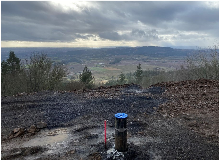
New well in NW Region
