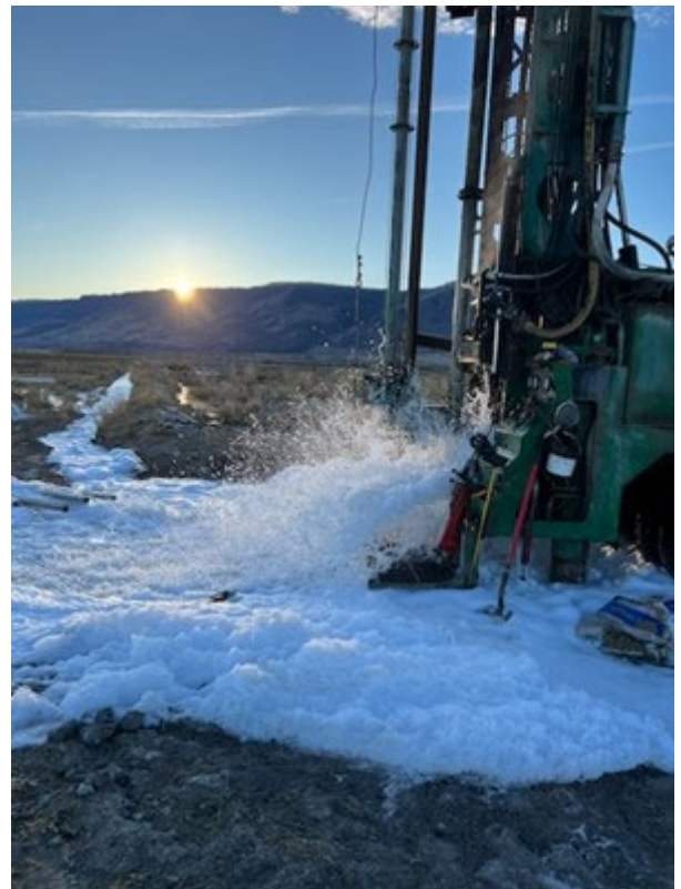
Drilling a well in south central Oregon.
