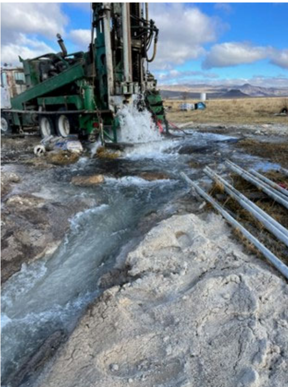
A flowing artesian well in south central Oregon
