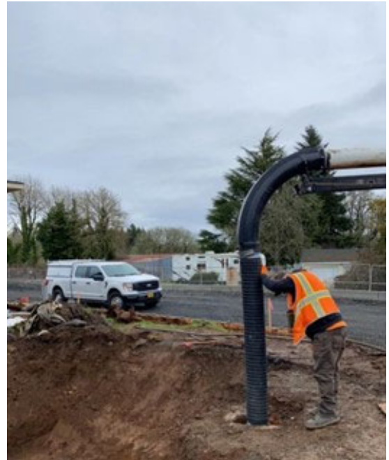
Dug well cleanout for abandonment
