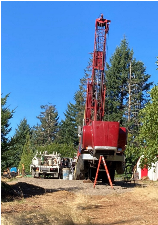
Drill rig in NW Oregon
