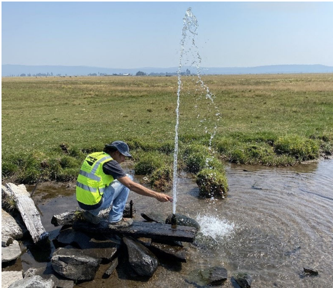
Improperly capped flowing artesian well
