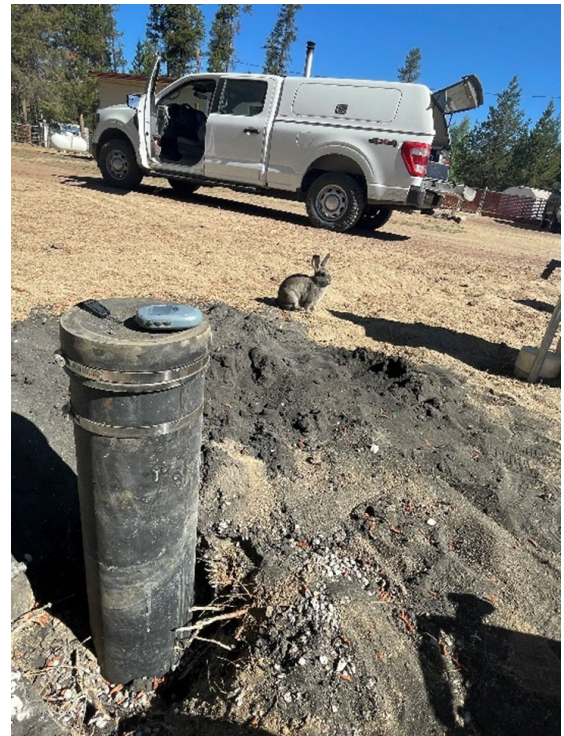
Wild rabbit helping inspect a well
