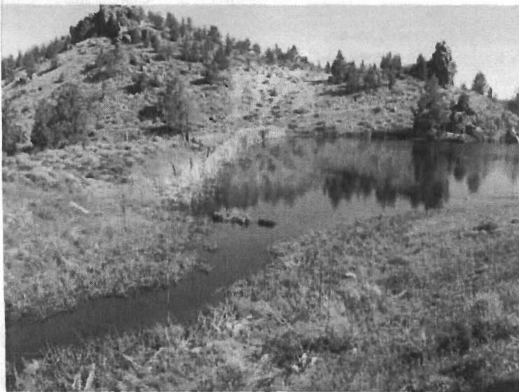
Spillway for Barnes Butte Dam
