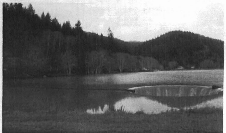
Drop Inlet Spillway for Fishhawk dam
