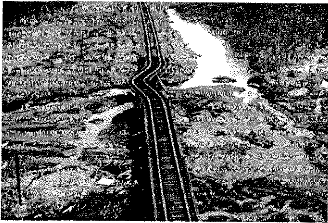
Transportation systems like railroads are fragile because a break in any spot can affect all traffic on the line. Ground response of loose, water-filled soils buckled this railroad bridge in the 1964 Alaska earthquake. Photo: USGS
