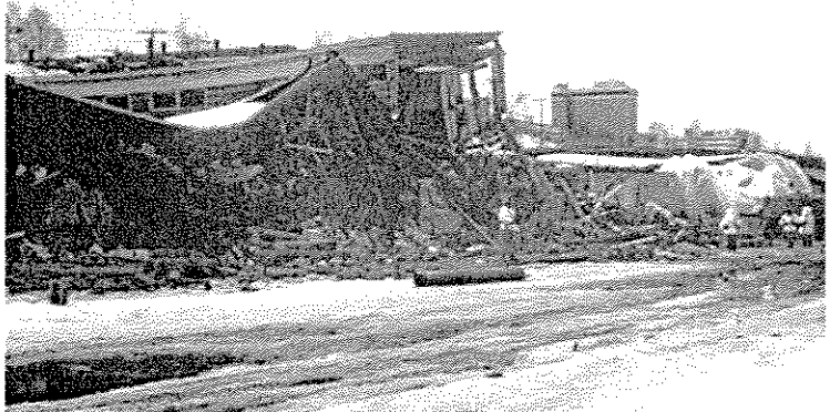
Warehouses at the toe of the Fourth Avenue landslide in Anchorage in 1964 were destroyed by compressional buckling and foreshortening. Much of the supply of food and drink for the city was stored in these buildings. Photo: USGS
