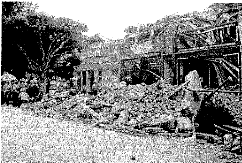
Debris from fallen buildings will trap people and make streets impassable. After the 1989 Loma Prieta, California earthquake, this group in Santa Cruz worked to rescue people. Photo: C. E. Meyer, USGS
