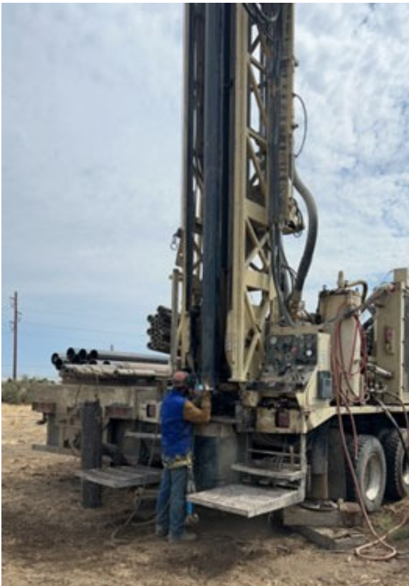
Well Constructor Welding Casing in Eastern Oregon
