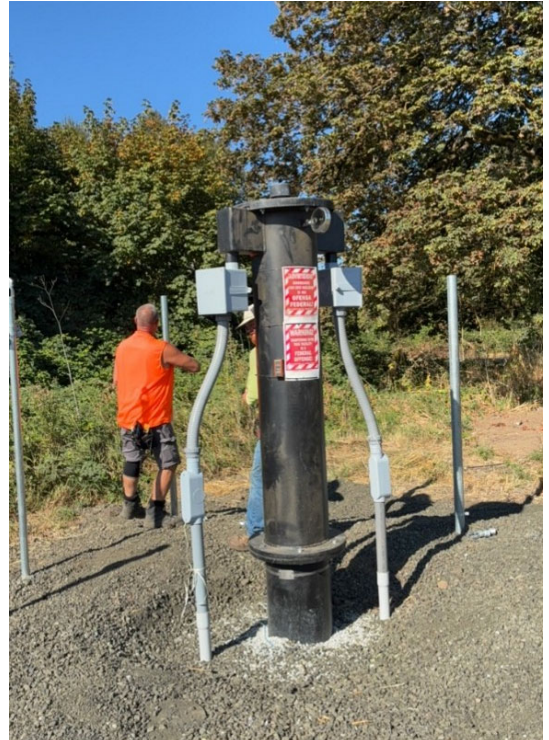
Raised Casing in the 100-Year Flood Zone
