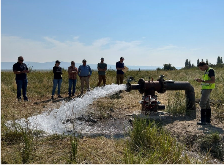
Flowing Artesian Well Inspection in Southern Oregon
