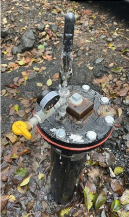
Improper flowing artesian well cap
