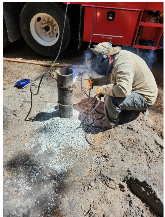
Well constructor welding casing
