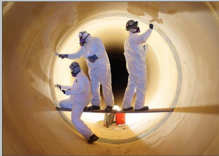
Lining pipe for COID's Juniper Ridge Project
