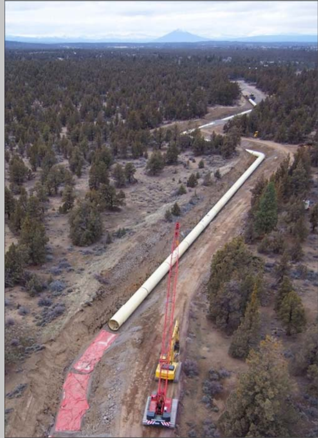
Laying pipe for COID's Juniper Ridge Project
