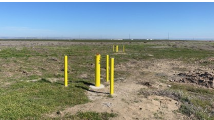
New monitoring wells in North Central Oregon
