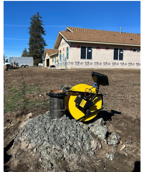
New well in South Central Oregon
