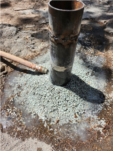
Bentonite being hydrated during seal installation
