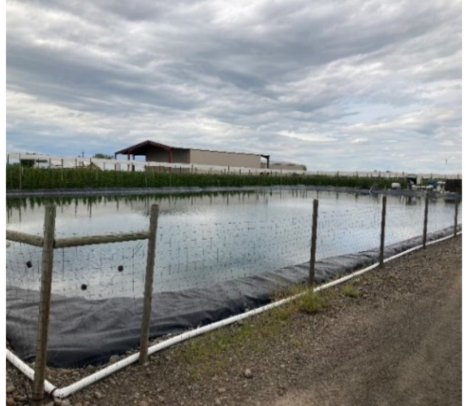
Example of a bulge in the system
